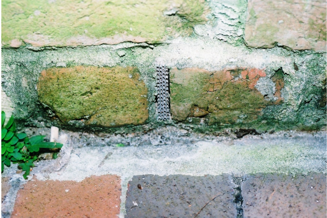
Photograph 9. A weep hole screen device in the mortar joint between bricks.
