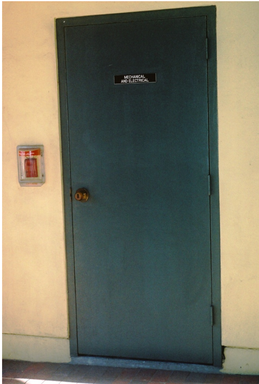
Photograph 7. A door leading to a mechanical area at the front of the carriage way.
