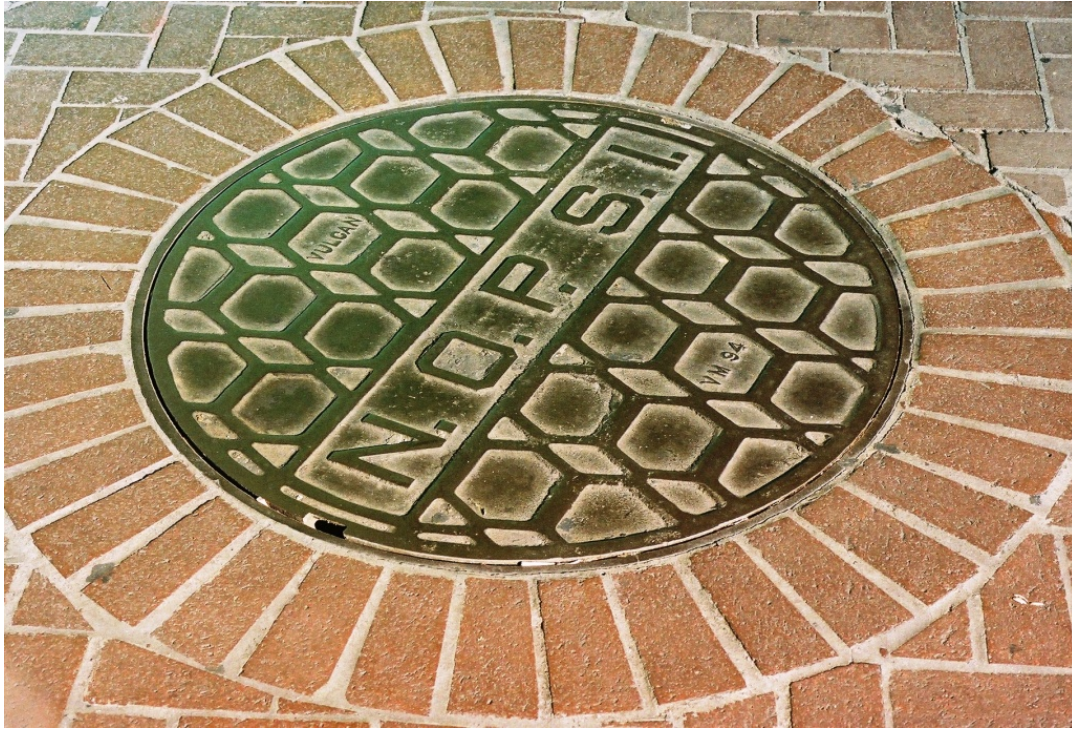
Photograph 5. A sewer manhole cover in the sidewalk immediately in front of the green doors leading to the building.
