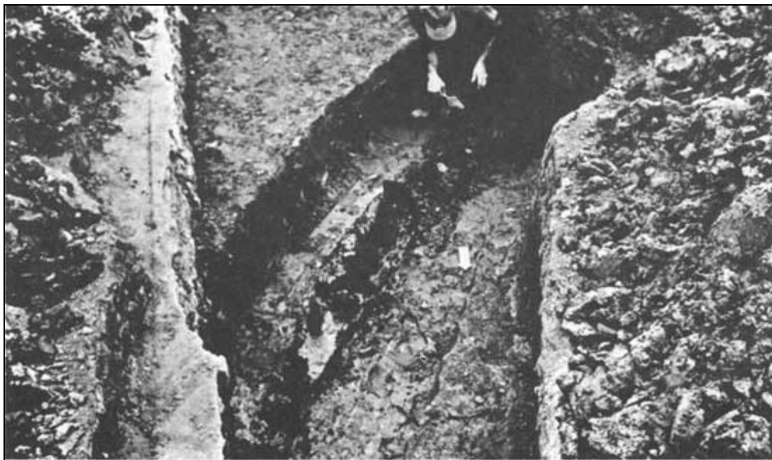
Fig. 18. Second section of water-preserved post ends (Trench "D-D").
