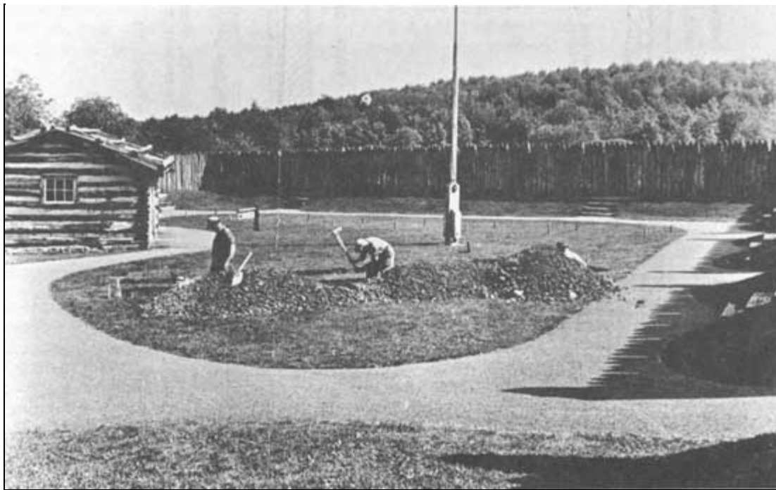
Fig. 15. Exploratory Trench "E" inside 1932 stockade.
