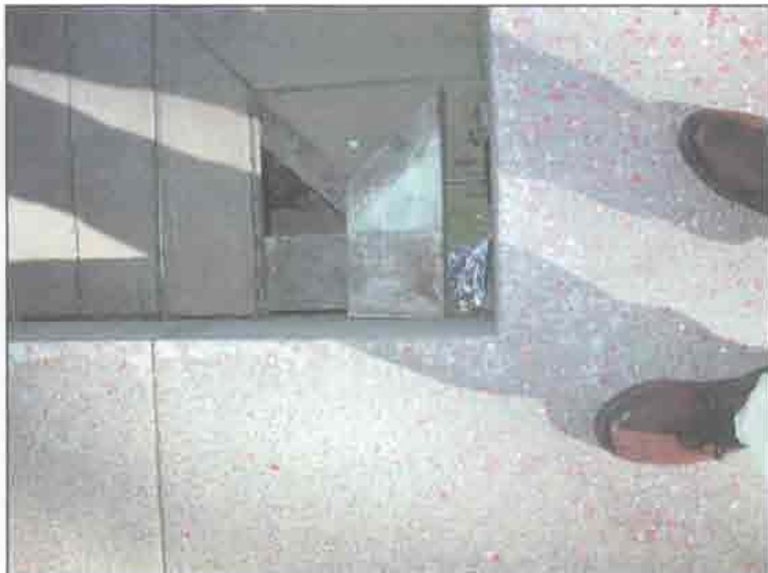
Condition Photo 14: Wood Walkway – Barrette Tier by Stair 1; Components are not properly fastened at wood walkway. (Courtesy of ARG, 2003)
