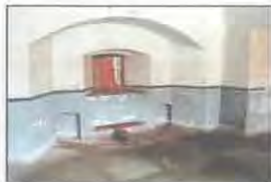
Typical cannon embrasure. This embrasure in casemate 2 still retains part of its original front pintle carriages. (John Martini, 2005)
