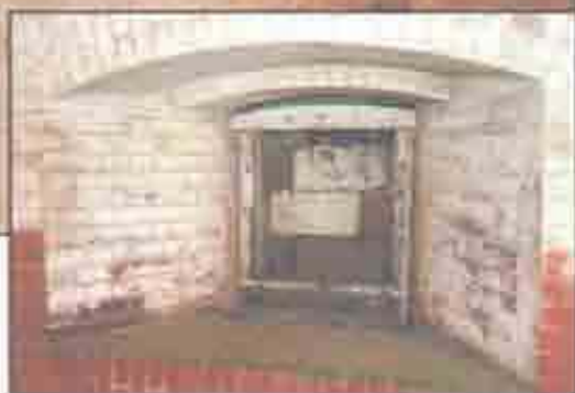
Most of the iron embrasures have deteriorated over the years and the openings have been infilled with brick and block for security purposes. (John Martini, 2005)
