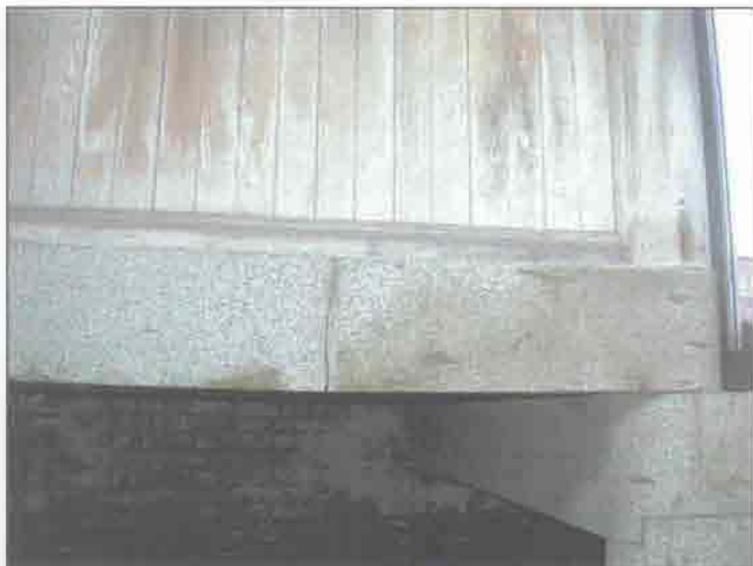
Condition Photo 6: Top Landing at Barbetta Tier; Crack in granite. (Courtesy of ARG, 2003)
