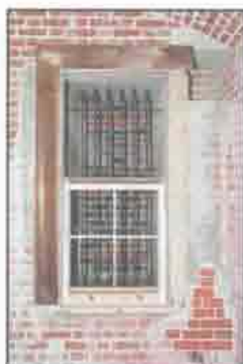
Rifle slit openings were enlarged and then bricked up leaving various building components. (John Martini, 2005)
