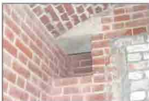
One of the square vents in the corner of each magazine with a small granite header. (John Martini, 2005)
