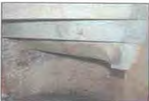
Stair #2 - Extra headroom was created between the 1st and 2nd tiers by carving into the granite tread. (John Martini, 2005)
