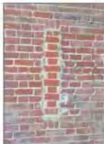
Former rifle slit on south flank filled in with brick. (Jane Lehman, 2005)
