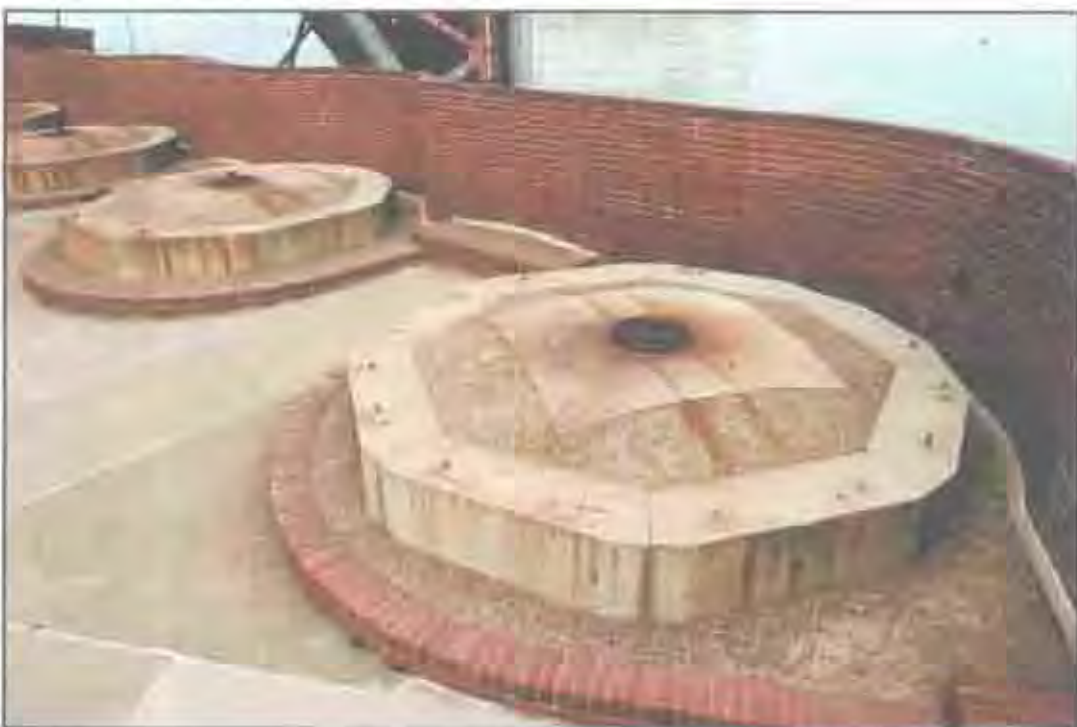
The octagonal cannon mounts on the barbette tier were designed to hold 10" columbiads. (John Martini, 2005)
