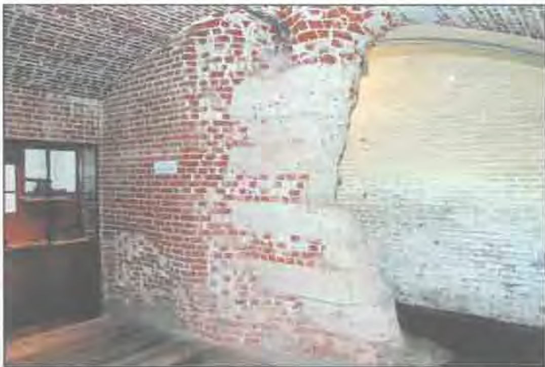
Walls were removed in the magazines during the conversion of the fort to a disciplinary barracks in 1914. Half of the 4-foot thick brick and rubble wall remains at right, while only the outline of a wall remains above. (John Martini, 2005)
