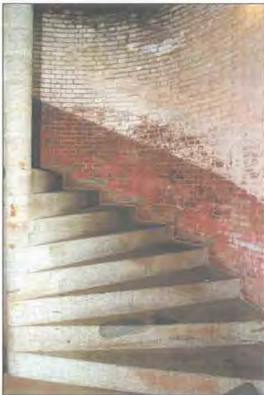
Typical interior of circular staircase showing curving brick walls and wedge-shaped granite treads. (John Martini, 2005)
