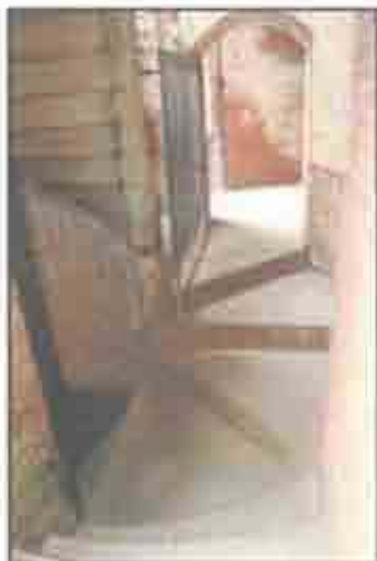
Each landing in the circular staircase is composed of slightly different shaped pieces of granite depending on the floor-to-floor heights. (John Martino, 2005)
