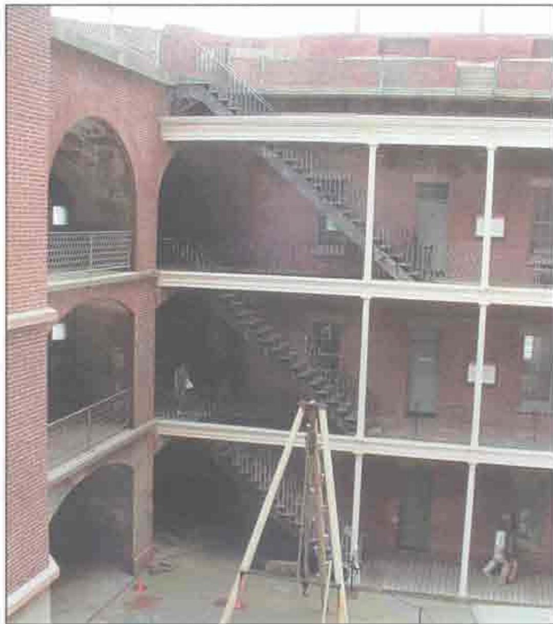
The cast iron staircase at the west end of the gallery is the only straight-run staircase in the fort. (Jane Lehman, 2005)
