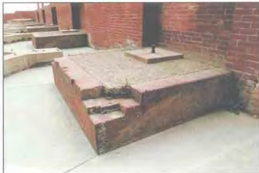
Along the southwest barbettes wall is a series of 11 platforms designed to hold 32-pounder guns. (John Martini, 2005)
