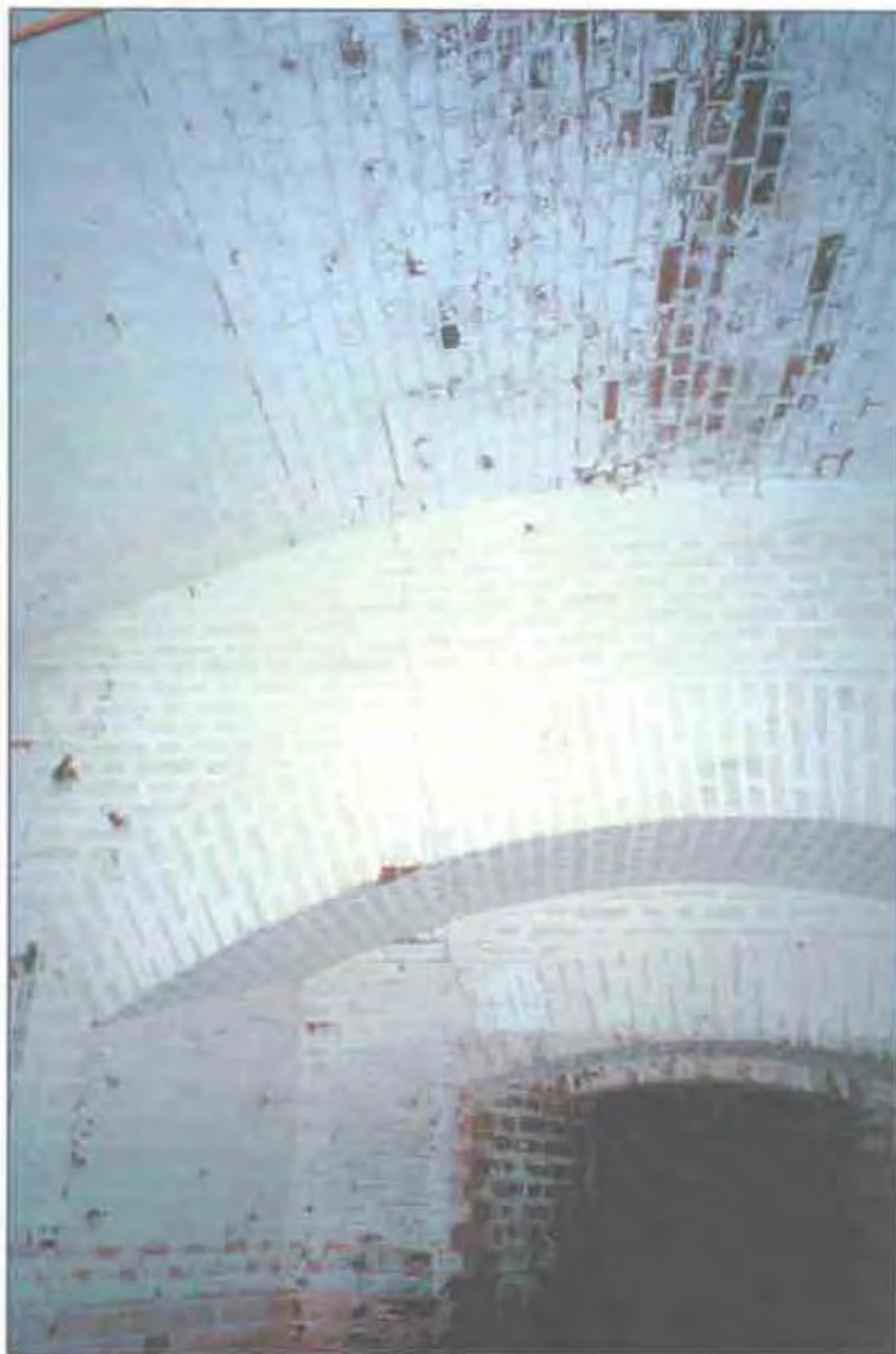
Condition Photo 15: Casemate 19: Cracks in brick masonry and joints have failed. The heavily flaking paint is typical in casemats. (Courtesy of ARG, 2003)
