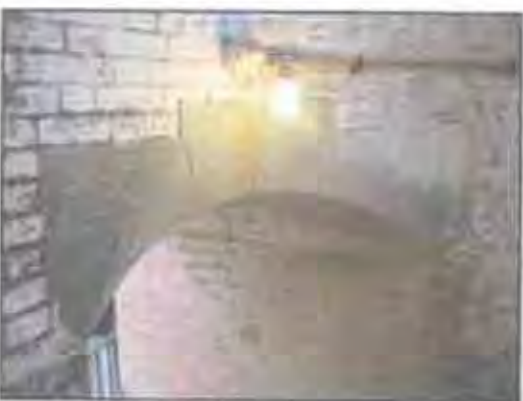
Stair #3 - The header over the openings on the 3rd tier consist of a 3-part segmental granite arch. (Jane Lehman, 2005)
