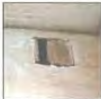
This 12" x 12" metal vent provides the only air circulation into the jail cells when the door was closed. (John Martini, 2005)
