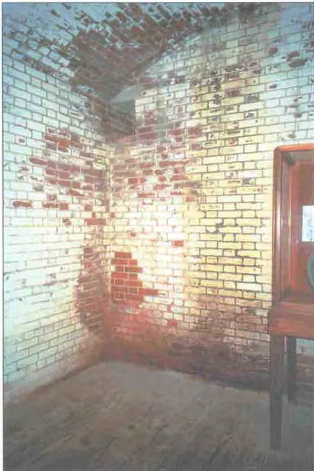
Condition Photo 16: Casemate 11. Open joints at the brick masonry and heavy water infiltration. Biological growth on the interior brick. (Courtesy of ARG, 2003).
