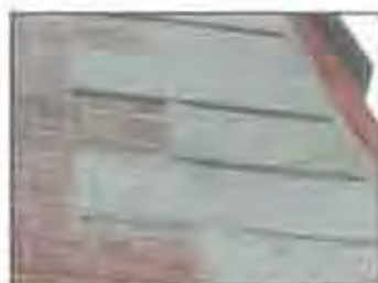
The quoins in the path of the wind and saltwater spray have lost their smooth quarried finish. (Jane Lehman, 2005)
