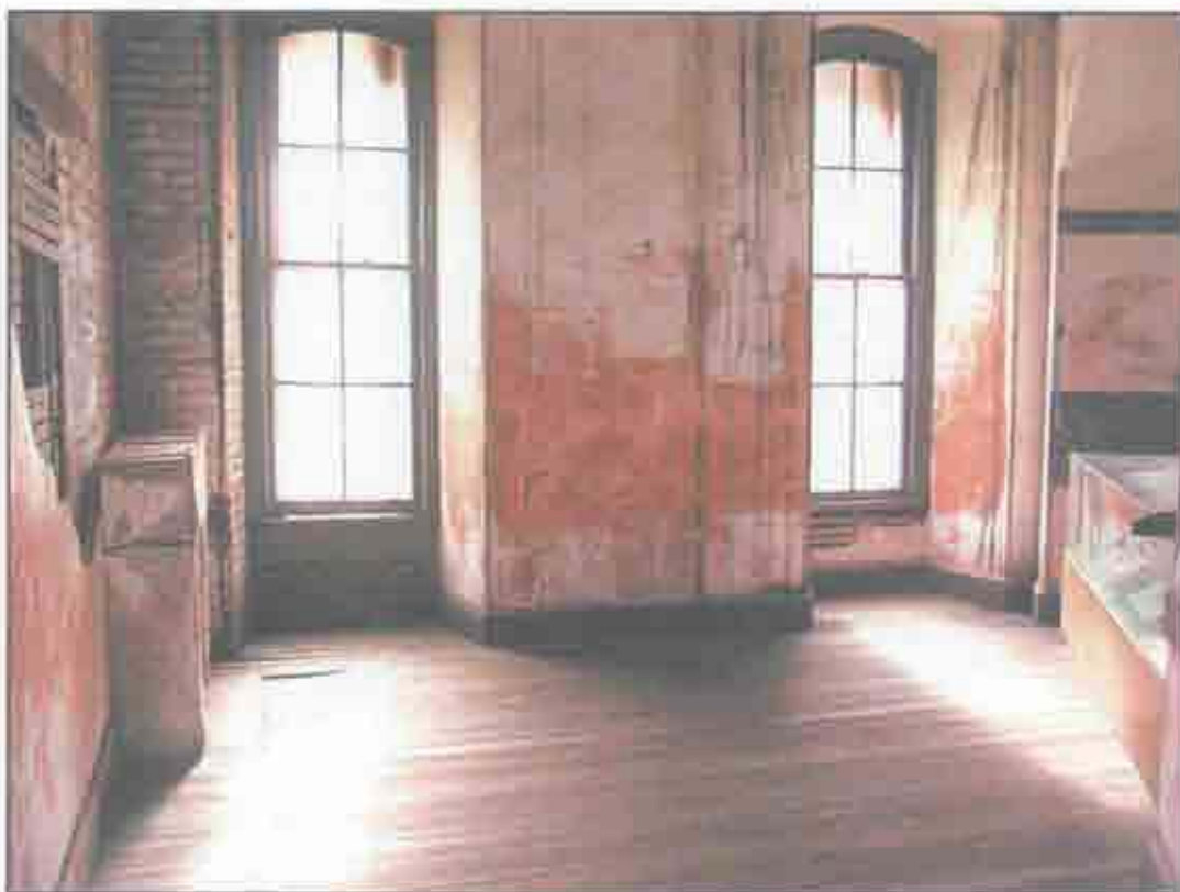
Condition Photo 23: Stained plaster at Casemate 21. (Courtesy of ARG, 2003)
