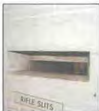
The rifle slit openings inside the guardroom measure 28" wide by 8" high. (John Martini, 2005)
