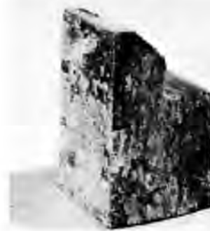
This small dentil was found between a floor joist and the wall in Independence Hall where it fell during a remodeling in 1815-16. The 51 mm x 32 mm fragment yielded clues to the size of the original room cornice and contained all paint colors applied to the woodwork.
