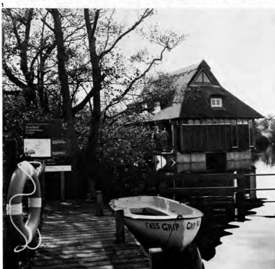
The Broadland Conservation Centre, Location, Design and Construction
