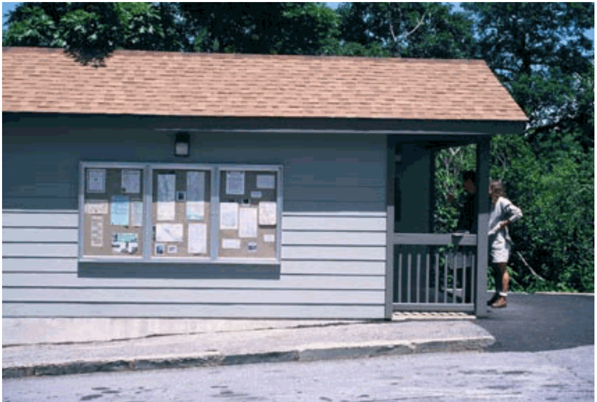
Figure 6: 2001 fee collection building (NPS).
