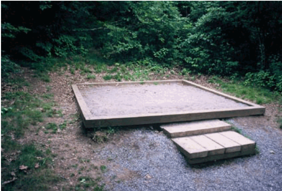
Figure 15: Typical level pad found at tent campsites (NPS).
