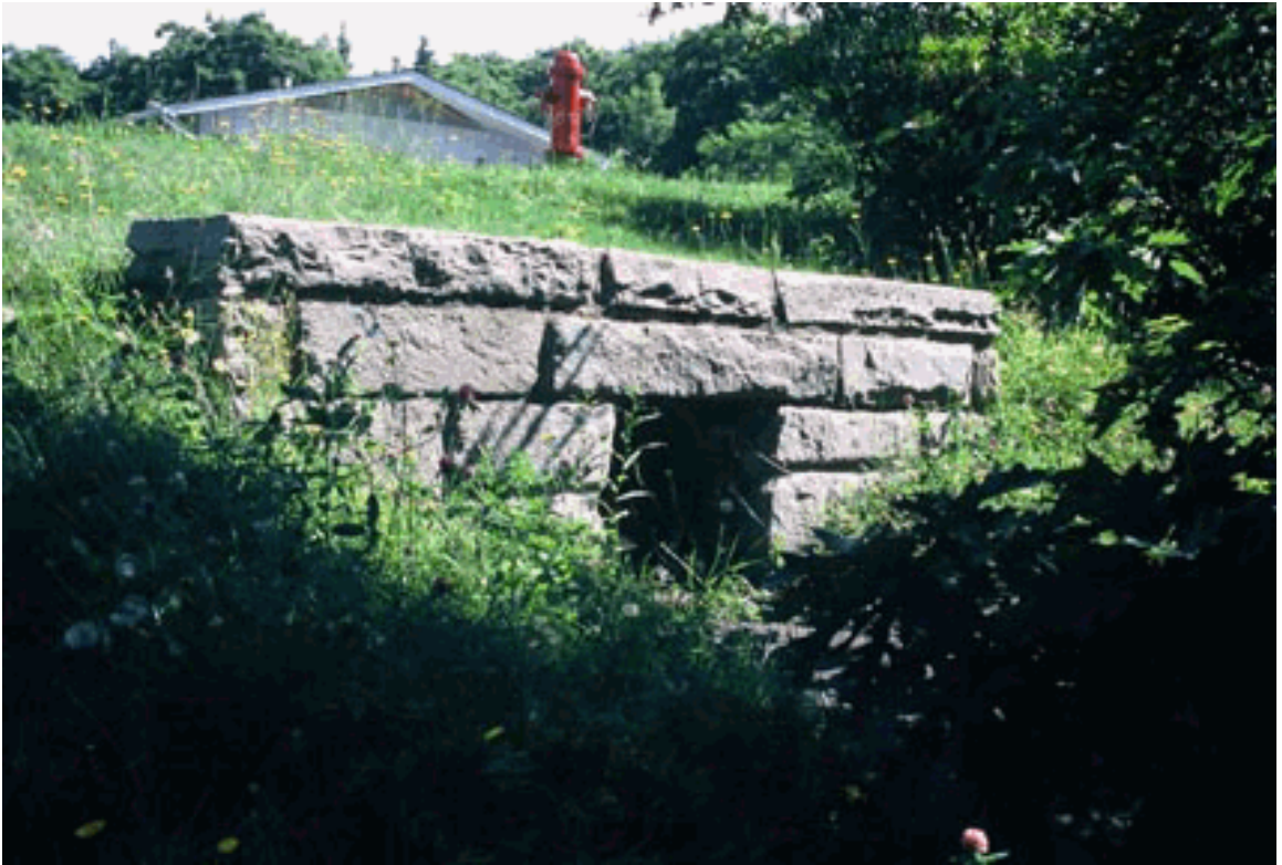
Figure 18: Stone head wall (NPS).
