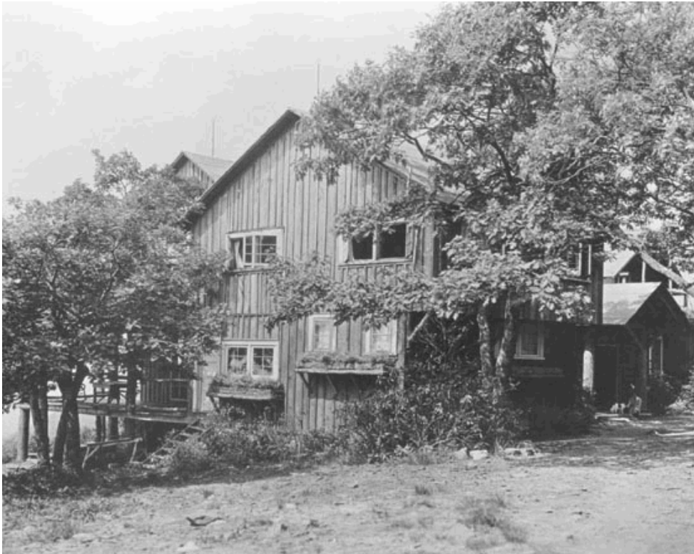
Figure 6: View of the Pisgah Forest Inn in 1923 (NPS).
