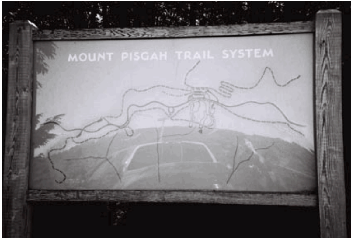
Figure 19: Sign featuring routed lettering and weathered wood posts (NPS).
