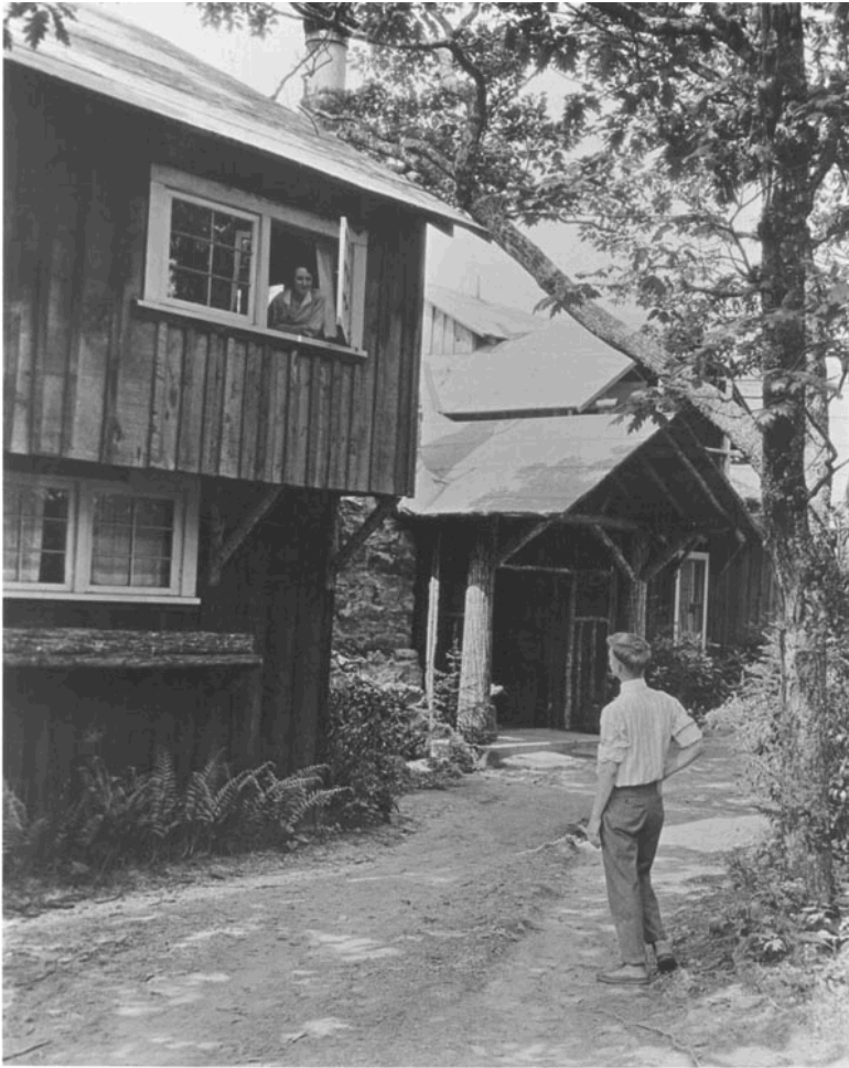
Figure 5: View of the Pisgah Forest Inn in 1923 (NPS).
