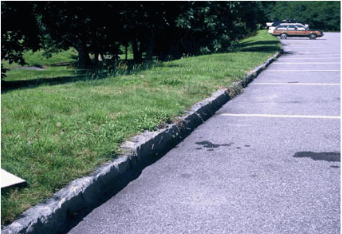
Figure 17: Stone curbing in the parking lot (NPS).
