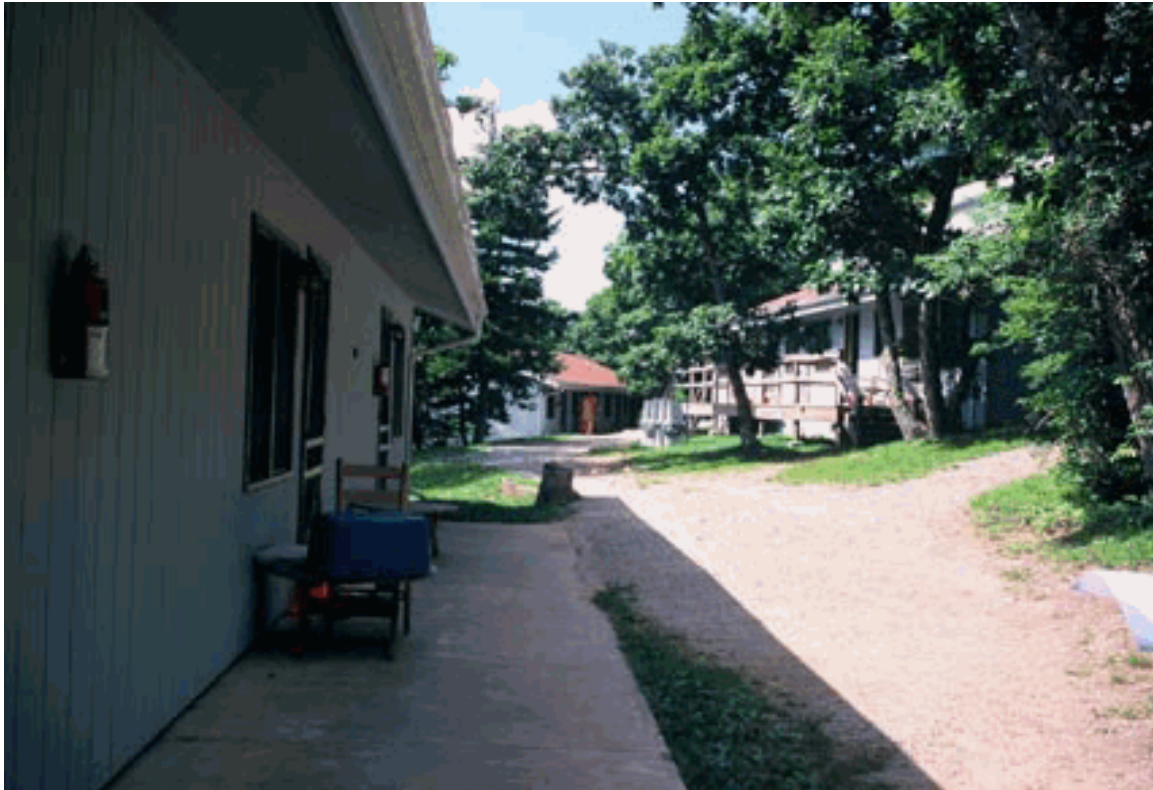
Figure 15: Employee dorms built in 1990 (NPS).
