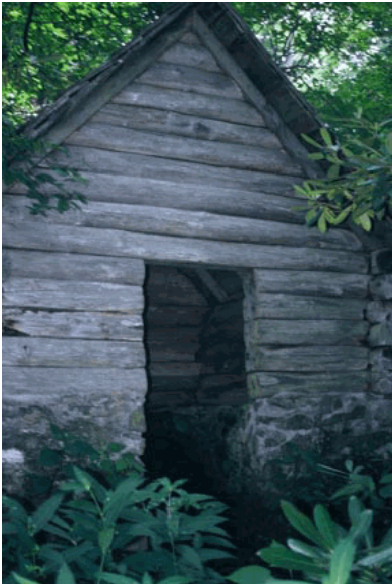
Figure 8: 2002 view of the front facade of the springhouse (NPS).
