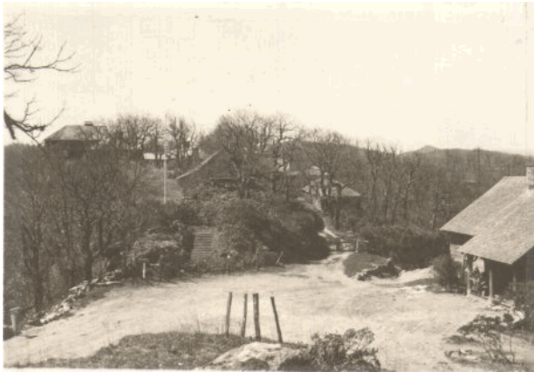
Figure 5: Buck Spring Lodge developed area (date unknown). Area in left foreground is the present day Buck Springs Overlook (NPS).
