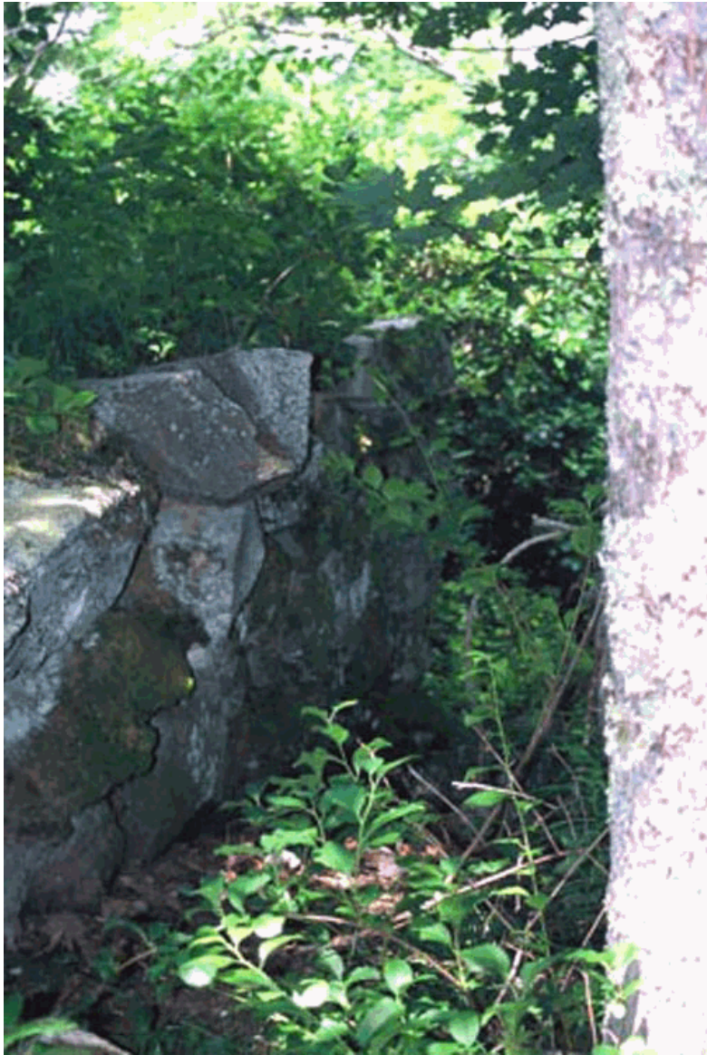
Figure 9: Portion of a stone wall that dates to the Vanderbilt era. These walls are now currently obscured by dense vegetation (NPS).
