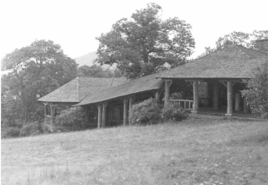
Figure 7: View of dining area and arcade to sleeping area with cleared grassed area in foreground, date unknown (NPS).
