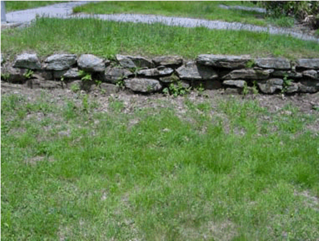
Figure 10: Historic stone retaining wall.
