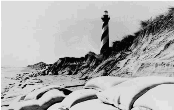
Sandbagging for erosion control (1968)
