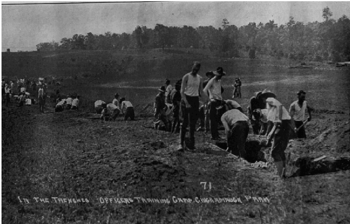
Digging trenches at Chickamauga Battlefield c. 1918. Photograph from CHCH archives, Camplife Magazines.
