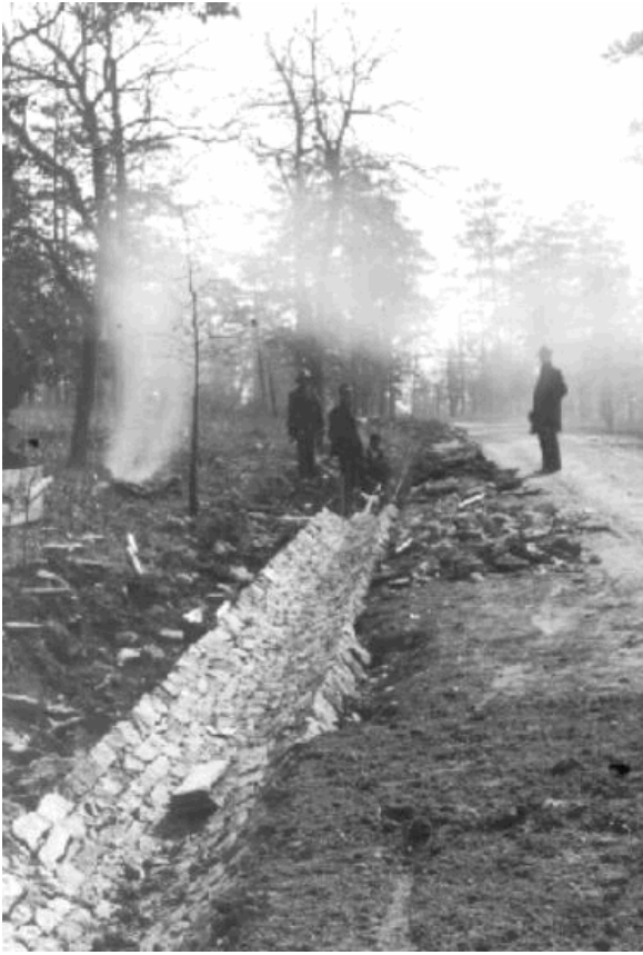
Road and drainage swale construction on Chickamauga Battlefield. Photograph from CHCH vertical files.
