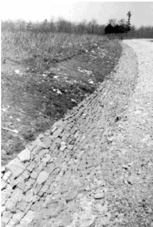
Roadside drainage swale at Chickamauga Battlefield.
