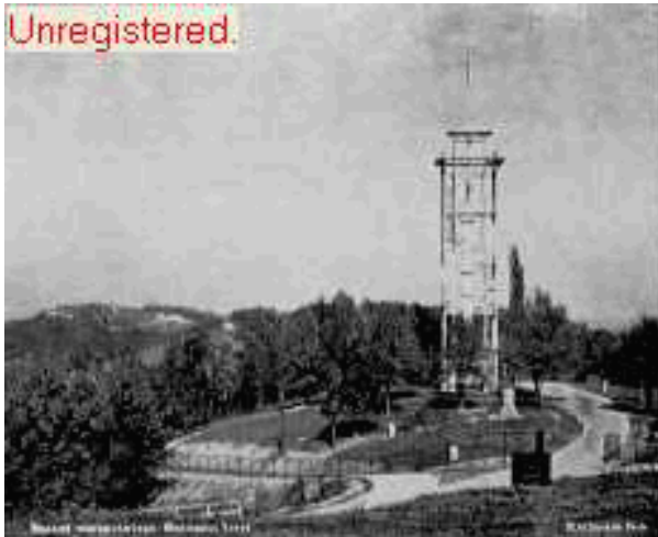
Looking north at Bragg Reservation. Note observation tower (non-extant) and commemorative landscape design, c. 1900.
