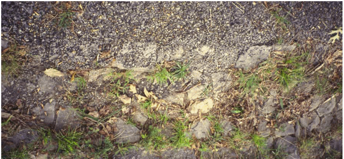
Contemporary view of stone-lined gutter along roadway at Orchard Knob.
