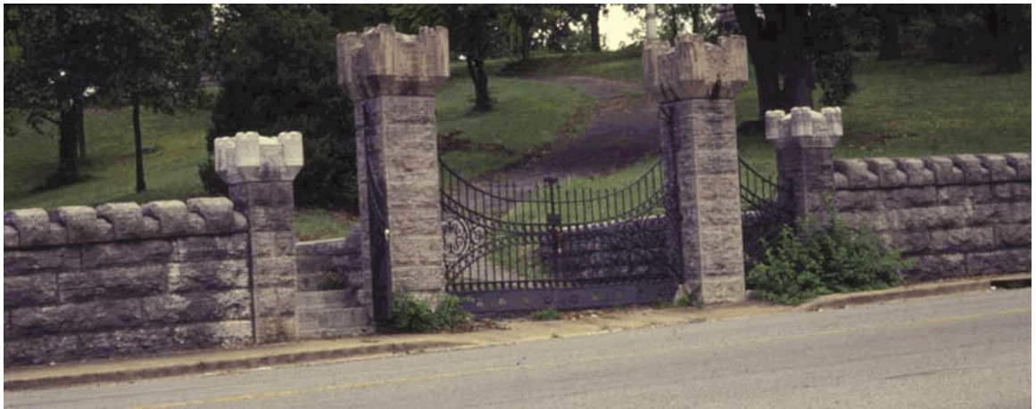
Entrance gate with crenelated walls and pathway leading up Orchard Knob.
