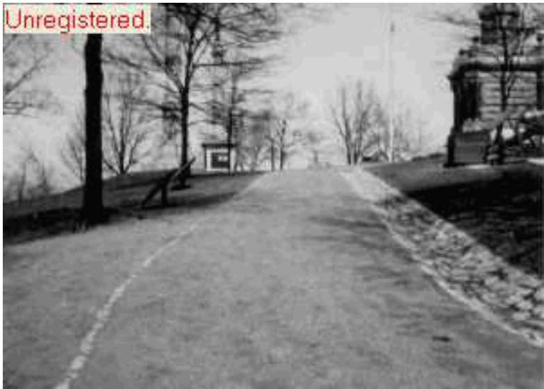
Orchard Knob after road improvements, c. 1935. Photograph from CHCH archives.
