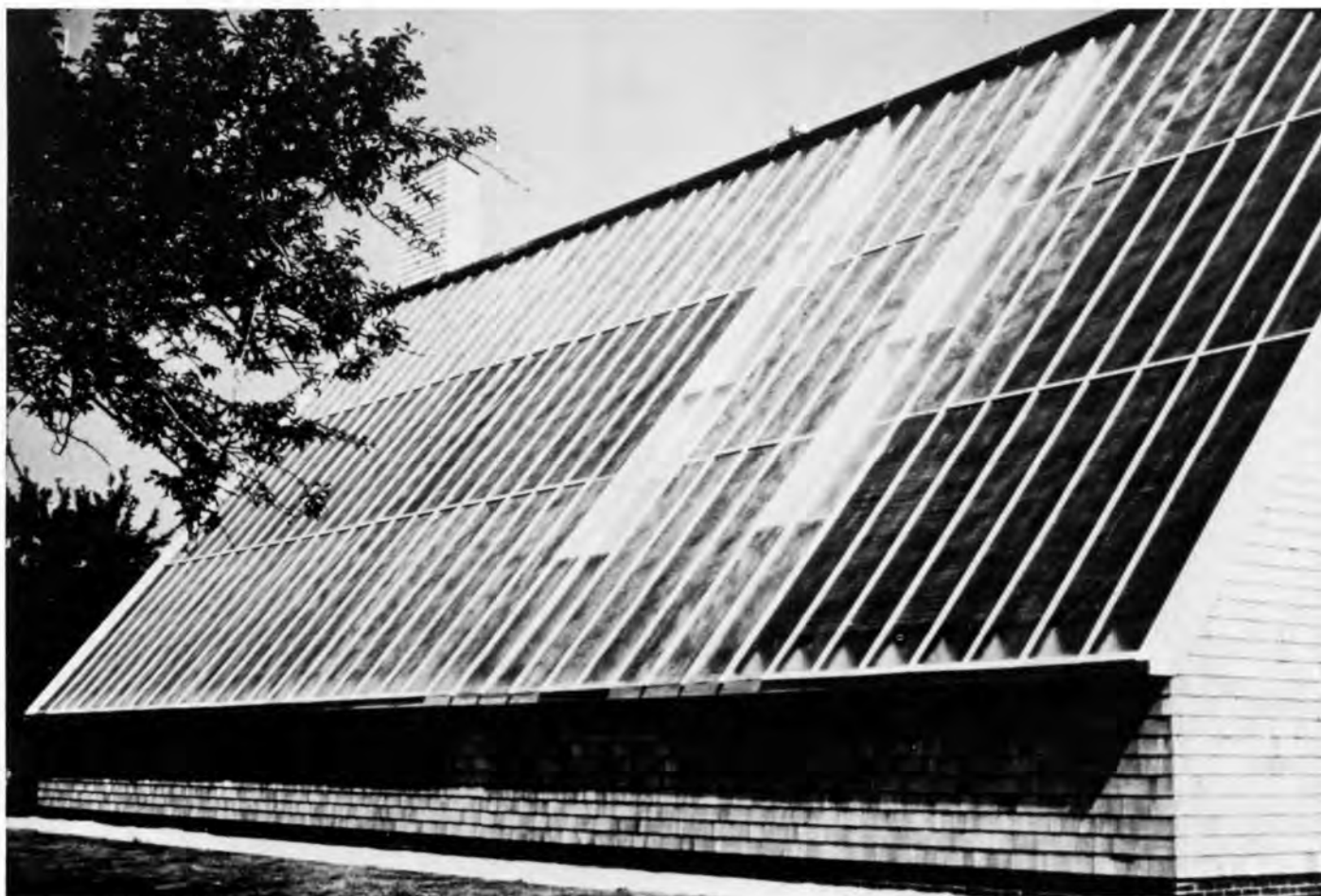
The south wall and roof of the Maine Audubon Society's headquarters building is composed almost entirely of solar collectors which are shallow troughs 2 feet (60 cm) wide. Heat is absorbed by black-painted screens and conveyed as hot air to a crushed rock storage bed. The 2000 square-foot (185.8 m 2 ) array can collect enough energy during 3 hours of sunlight to heat the building for 24 hours. Photo: Maine Audubon Society
