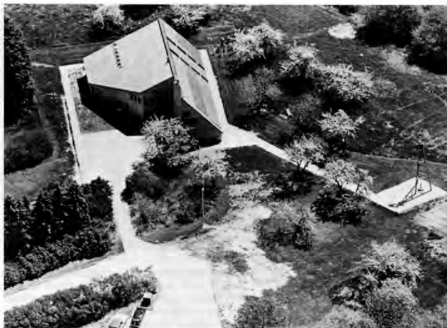
Aerial view of Gilsland Farm, looking east. Several siting considerations are visible including the relationship between the 2,000 square-foot ( 185.8\text{m}^2 ) southern collector face and the tapered north wall. Also on the north side, note the sloping roof and edge of the windbreak.
