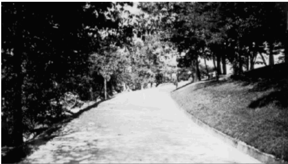
Completion of trail construction, c. 1935. Photograph from CHCH archives.
