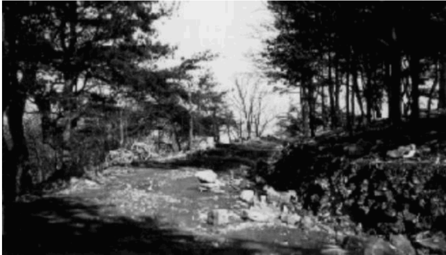
Trail construction at Point Park, c. 1935. Photograph from CHCH archives.
