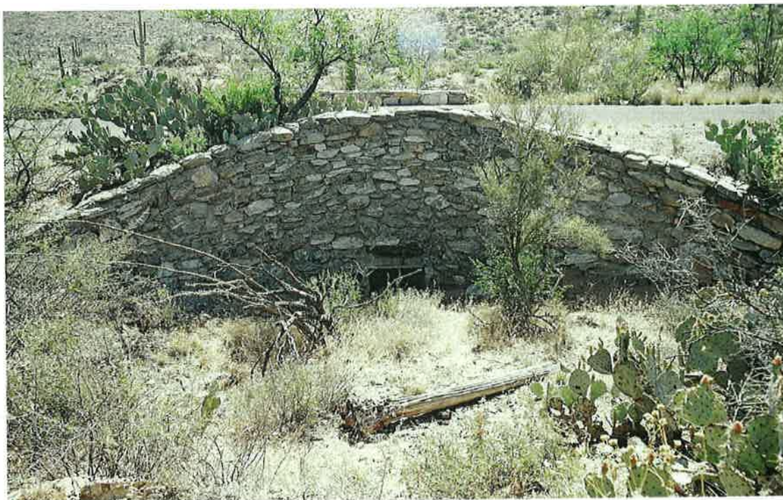
FIGURE 45. INTAKE CULVERT HEADWALL – DISCHARGE HEADWALL IN BACKGROUND
