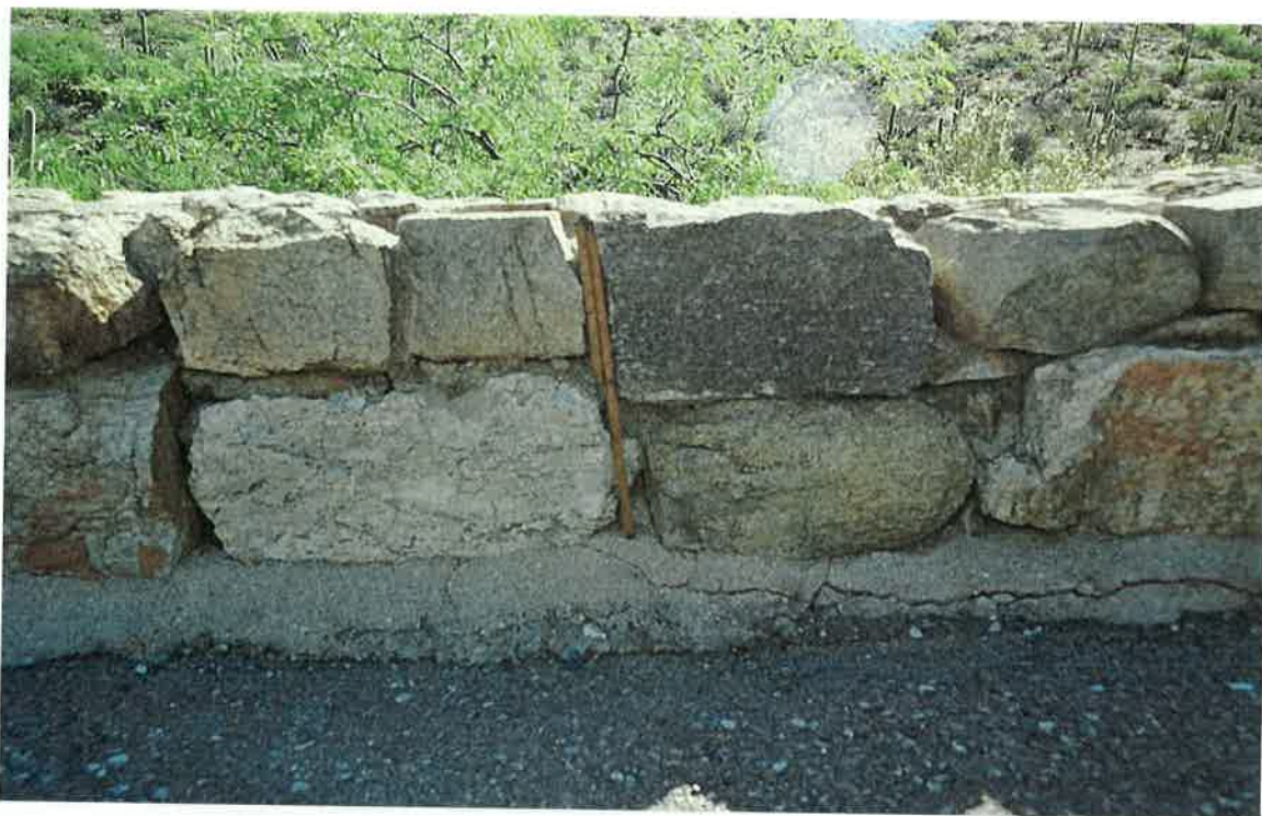
FIGURE 26. EXAMPLE OF WALL CONSTRUCTION, ROCK / COBBLE-SIZE VIEW FROM EXISTING ROADBED (NOTE THE NON-CCC CEMENT PATCHING ALONG BASE OF ROCK ALIGNMENT)
