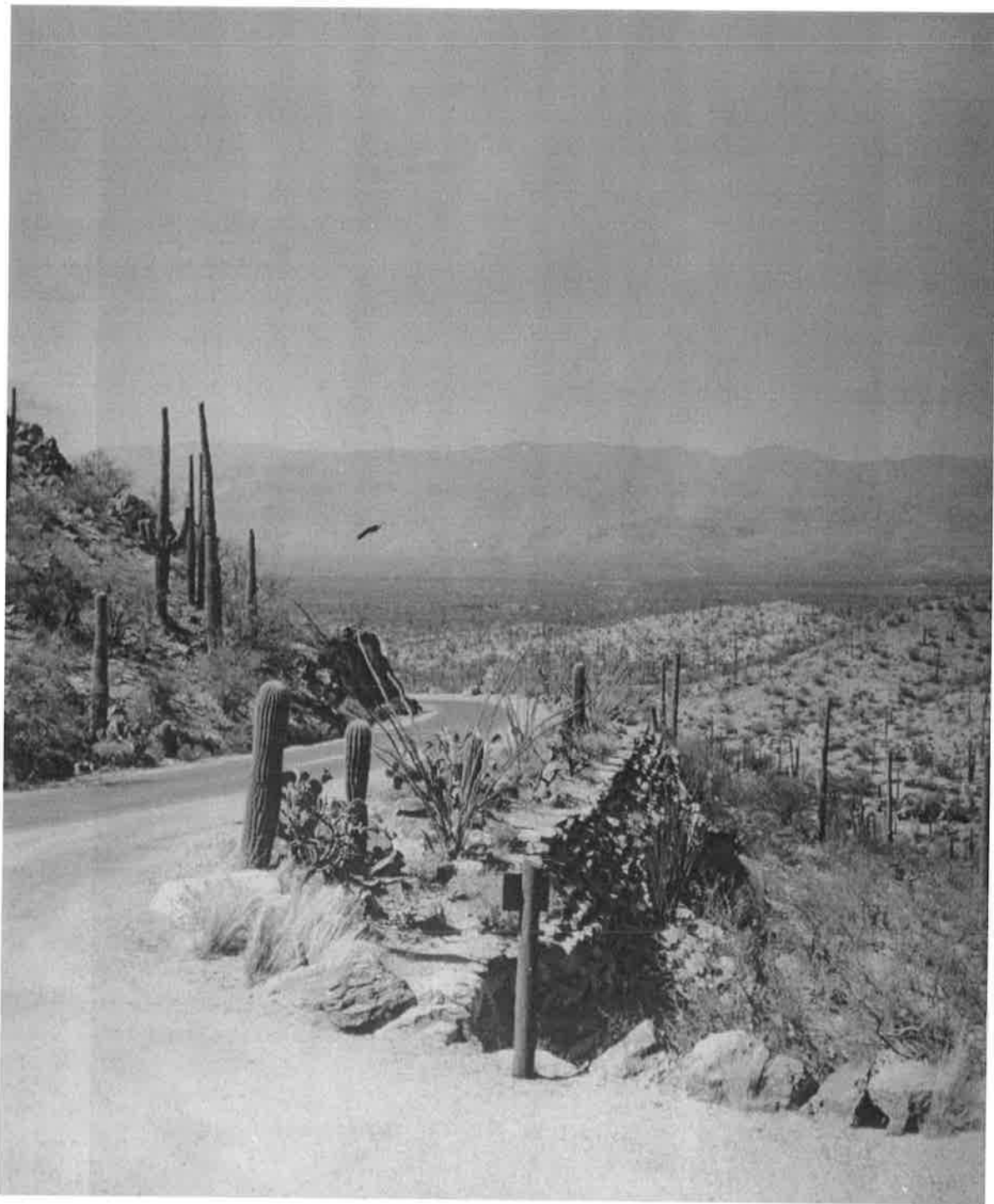
FIGURE 34. HISTORIC PHOTO (CA. 1950s) SHOWING WALL CONSTRUCTION AND GENERAL SETTING (SAME SETTING AND CONFIGURATION AS FIGURE 11)
