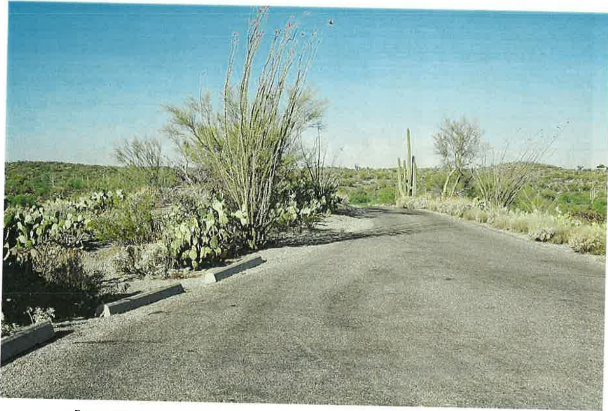
FIGURE 21. EXISTING CEMENT STOPS IN TURNOUT (LOOKING WEST FROM THE TURNOUT)
