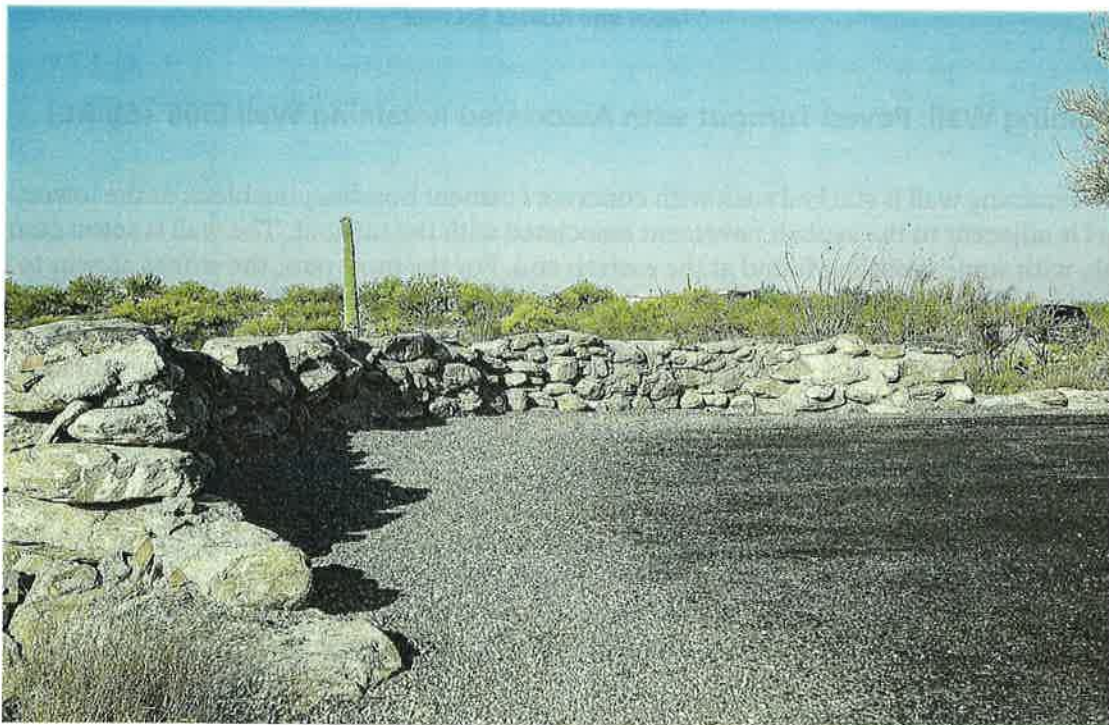
FIGURE 18. CLOSE UP OF WALL CONSTRUCTION AND ASSOCIATED TURNOUT
