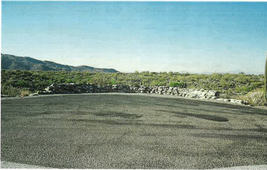
FIGURE 17. VIEW LOOKING SOUTH OF THE TURNOUT AND ASSOCIATED RETAINING WALL
