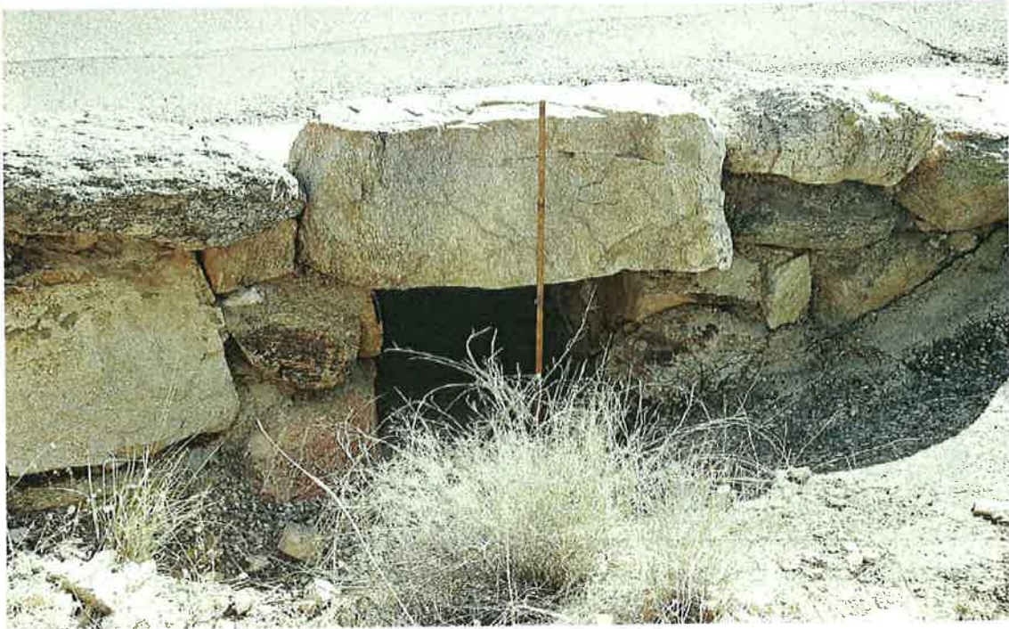
FIGURE 41. INTAKE CULVERT HEADWALL – STACKED ROCK WITH ASSOCIATED INTAKE BOX—CEMENT CULVERT RUNS UNDERNEATH THE EXISTING ROADBED
