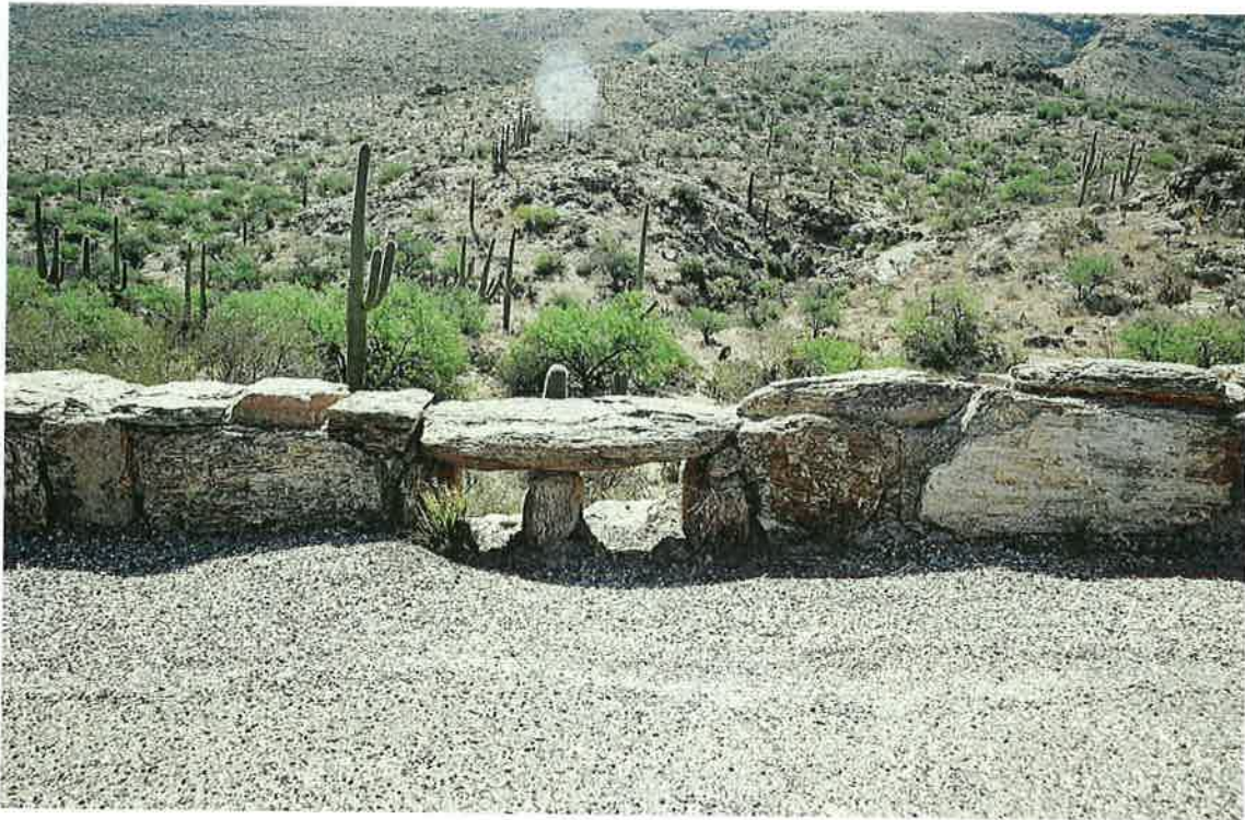
FIGURE 31. CLOSE UP OF BUILT-IN WATER DRAINS IN WALL—THIS PORTION OF WALL IS ONE LAYER HIGH WITH FLAT CAPSTONES
