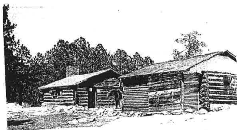
Manning Camp Ranger Station - elevation. approx. 8000 feet.
