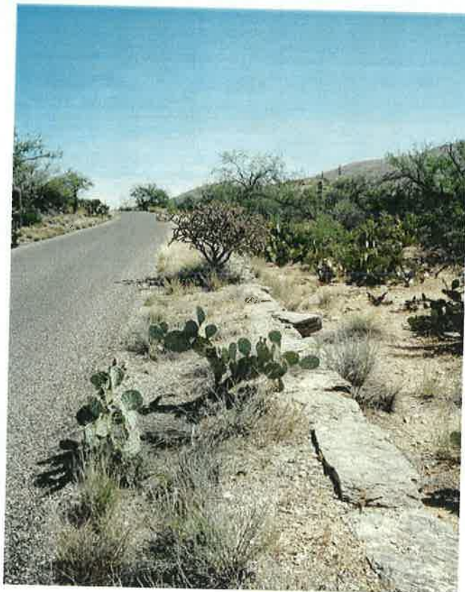
FIGURE 37. VIEW OF ROCK ALIGNMENT ALONG ROAD SHOULDER; TOP COURSE OF ROCK RESEMBLES CAPSTONE FOUND ON THE LARGER RETAINING WALLS
