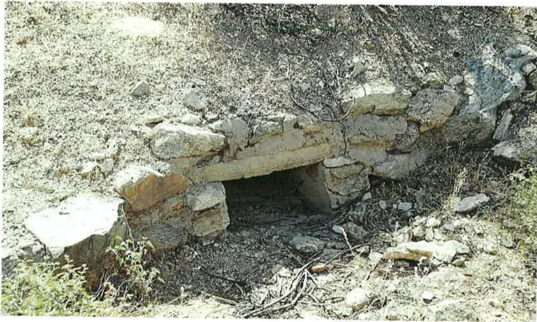
FIGURE 43. DISCHARGE CULVERT HEADWALL; DEFINED CEMENT CHANNEL THAT RUNS UNDER THE EXISTING ROADBED; MINIMAL STACKING
