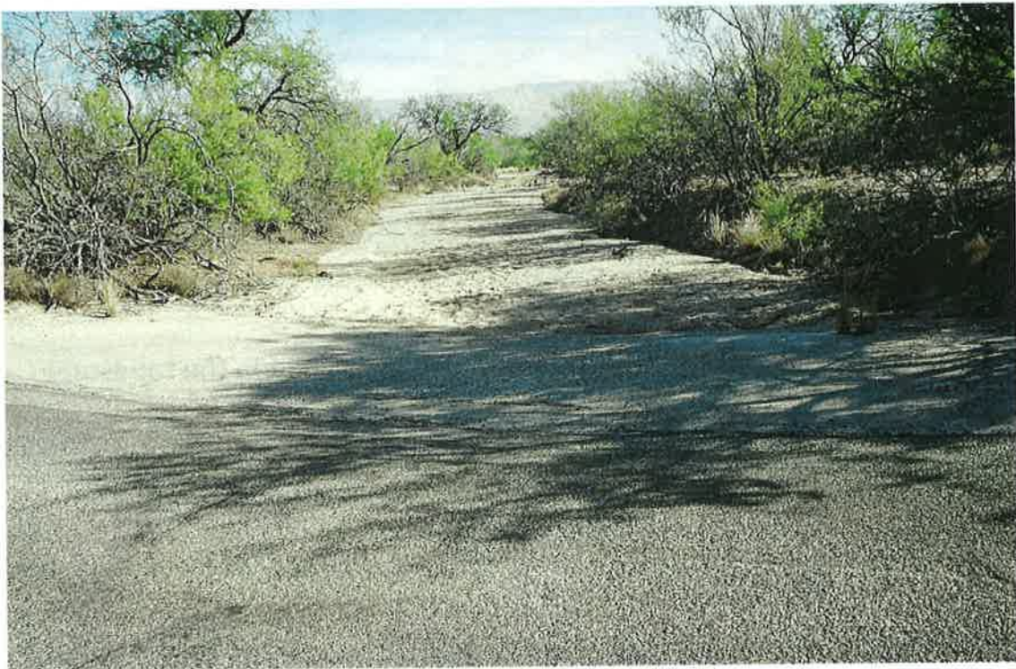
FIGURE 52. CLOSE-UP OF LOW-WATER CROSSING
