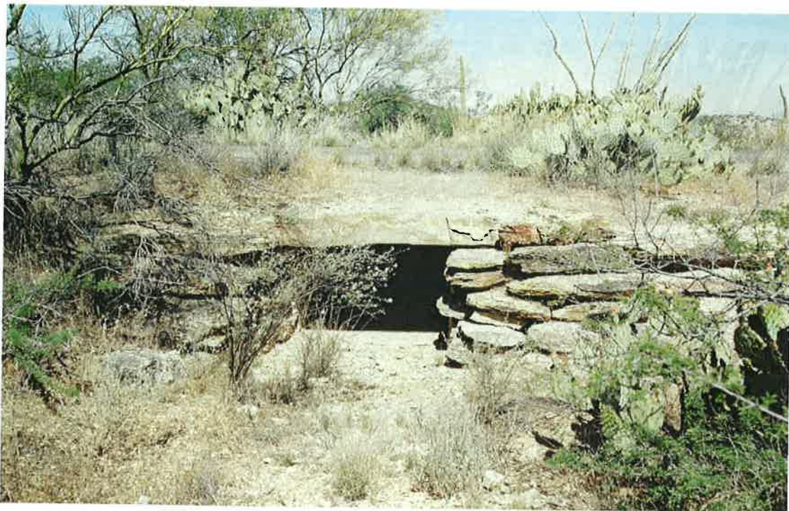
FIGURE 48. STACKED INTAKE CULVERT HEADWALL WITH CAPSTONE AND CEMENT CHANNEL
