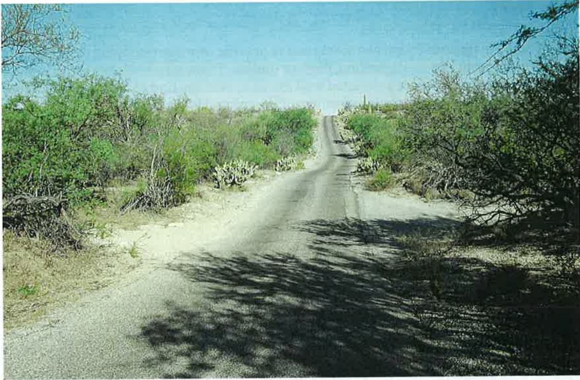
FIGURE 51. VIEW OF LOW-WATER CROSSING LOOKING FROM TURNOUT 506 + 60
