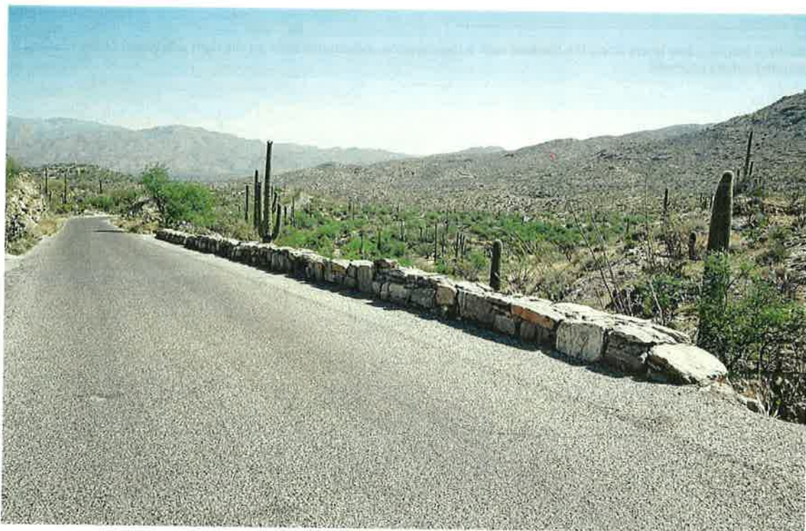
FIGURE 32. VIEW OF ROADBED AND END WALL LOOKING SOUTH
