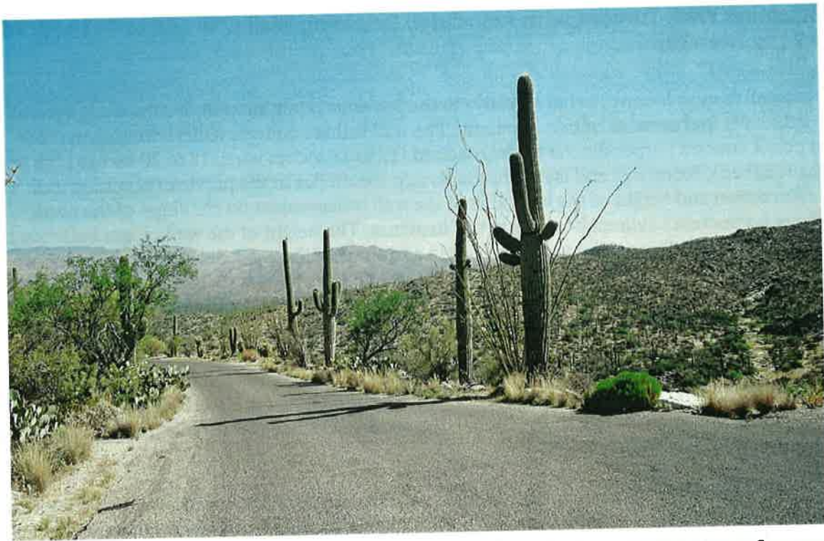
FIGURE 28. SEGMENT 4 – VIEW OF ROADBED LOOKING NORTH (DOWNHILL) – RETAINING WALL IS NOT SEEN FROM ROAD; BACK SIDE OF WALL IS 4 M TO 8 M IN HEIGHT (12 FT. TO 24 FT.)
