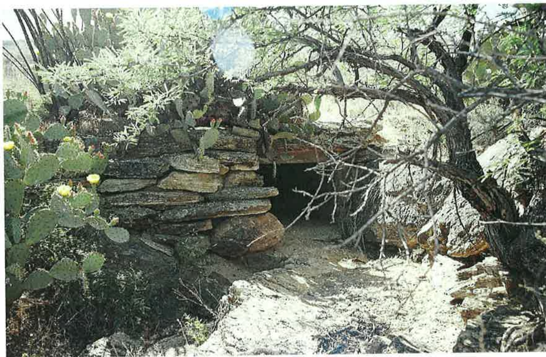
FIGURE 46. STACKED DISCHARGE CULVERT HEADWALL
