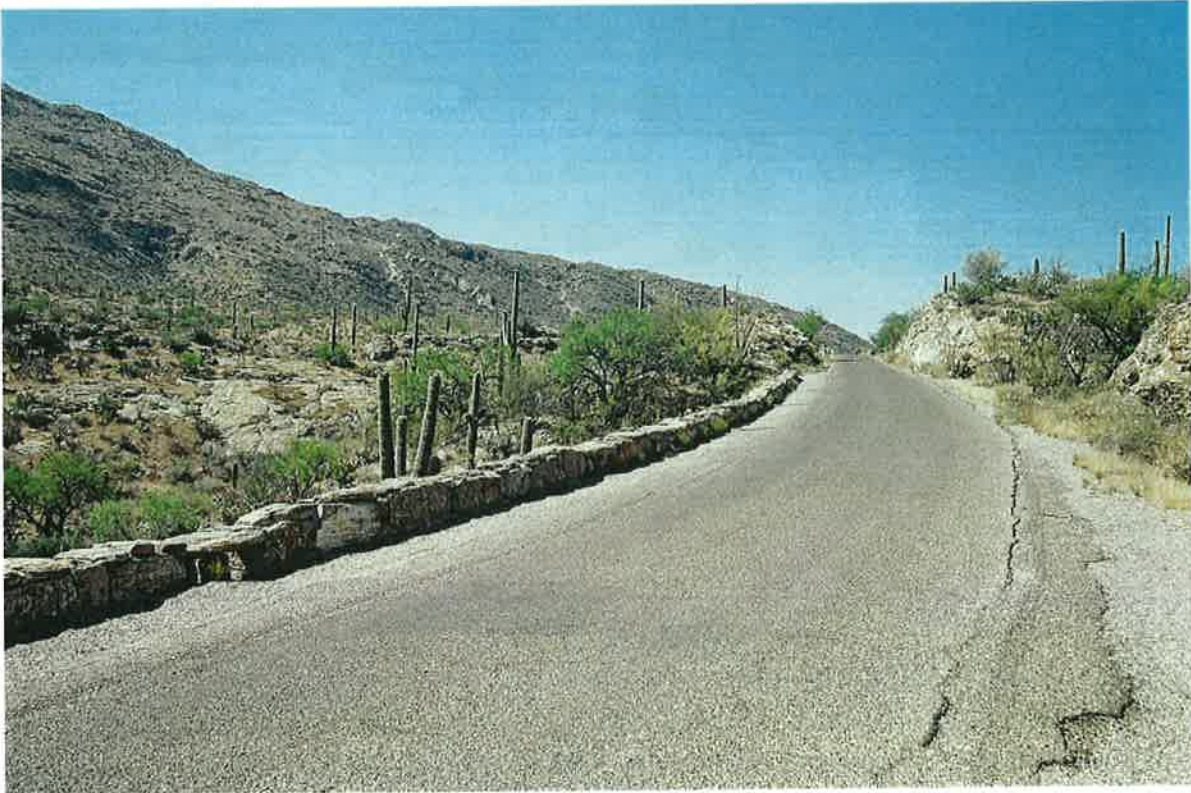
FIGURE 30. EXPOSED WALL ALONG SEGMENT 1 (740 + 05 TO 741 + 78) LOOKING NORTH
