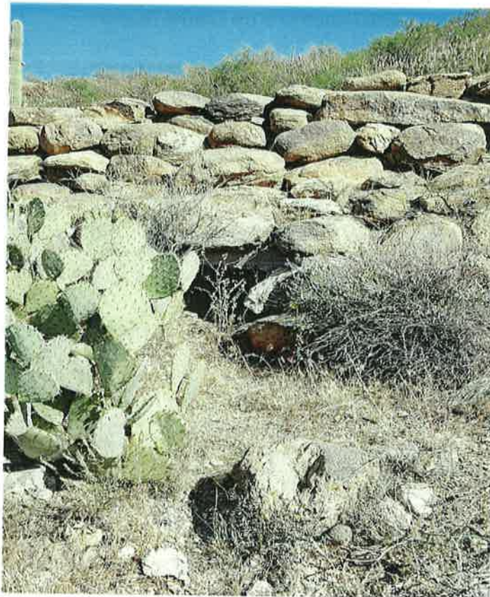
FIGURE 44. INTAKE CULVERT HEADWALL – ASSOCIATED STACK ROCK FEATURE, 5-6 COURSES HIGH
