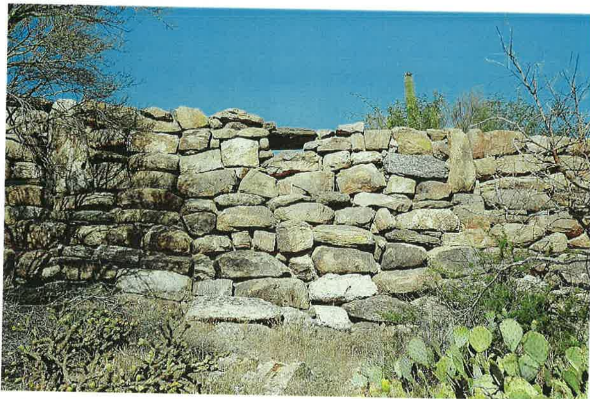
FIGURE 24. SEGMENT 2 – BACK SIDE OF WALL, DRAINAGE FEATURE CAN BE SEEN IN TOP PORTION OF PHOTO
