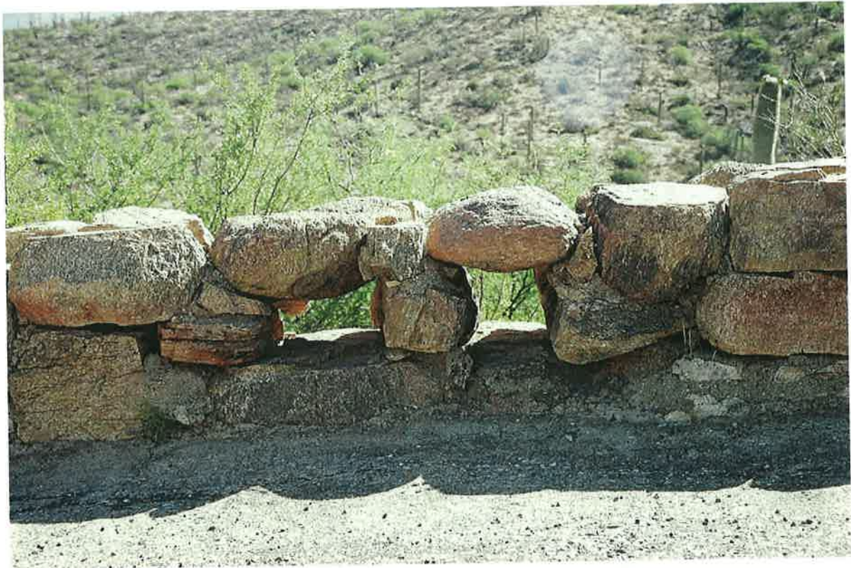
FIGURE 25. CLOSE-UP OF STONE CAPPING AND WATER CONTROL FEATURE BUILT INTO RETAINING WALL
