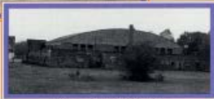
Hangar No. 1 (Rear View)
