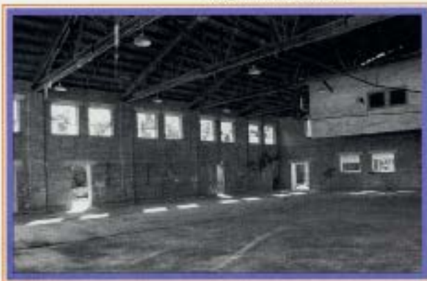
Interior, Hangar No. 1
