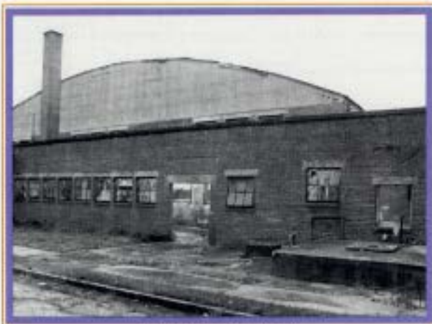
Moton Field, Hangar No. 1
