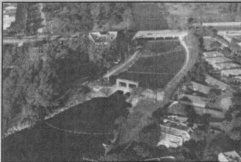
Figure 4. Flood control structure.
