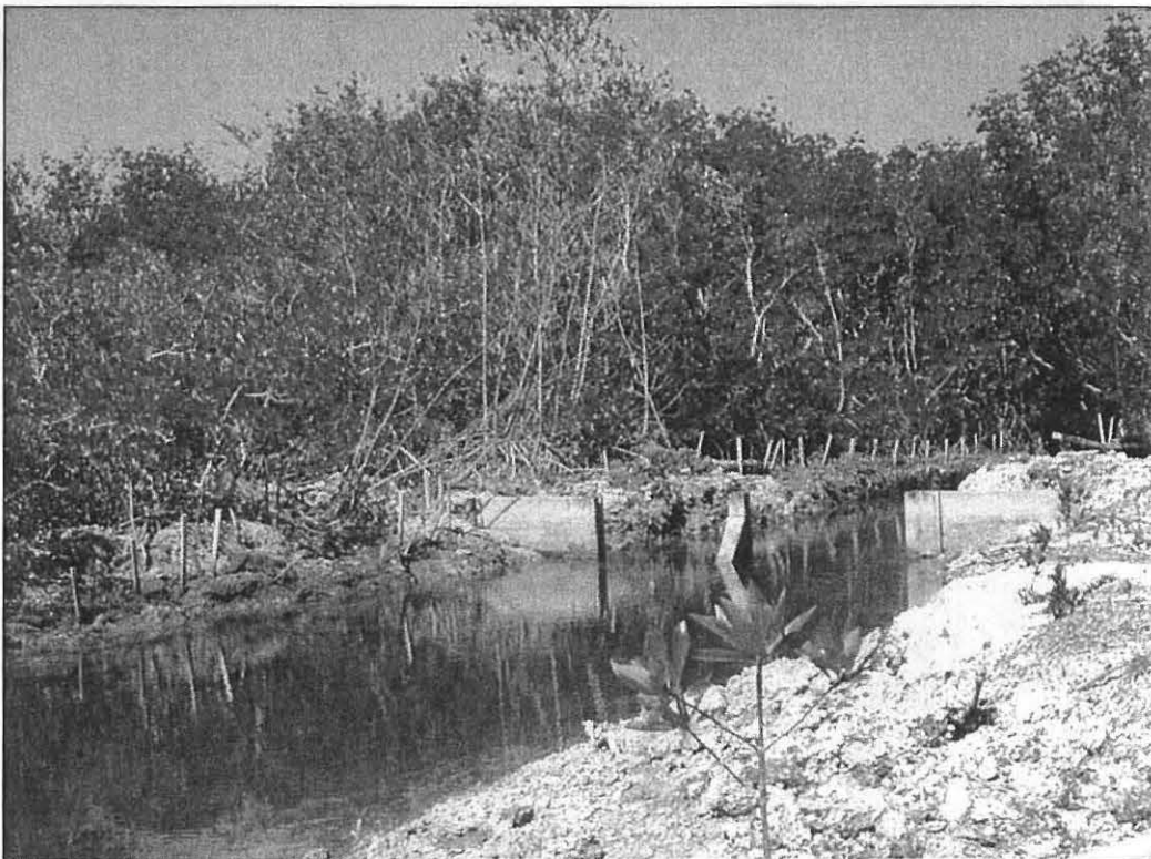
Photo 6: Reinforced adjustable weir at the north connection point. Outgoing tide.
