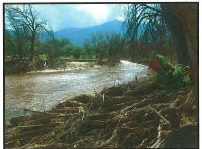
View looking upstream at large tributary showing erosion and channel widening.
