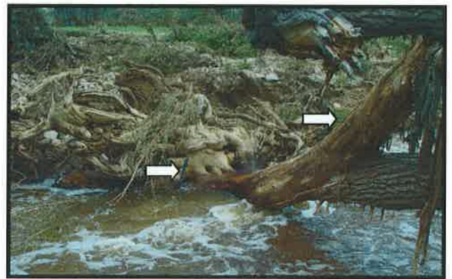
Transect 2. Only remnants of the staff gage and crest gage support structures remain.
