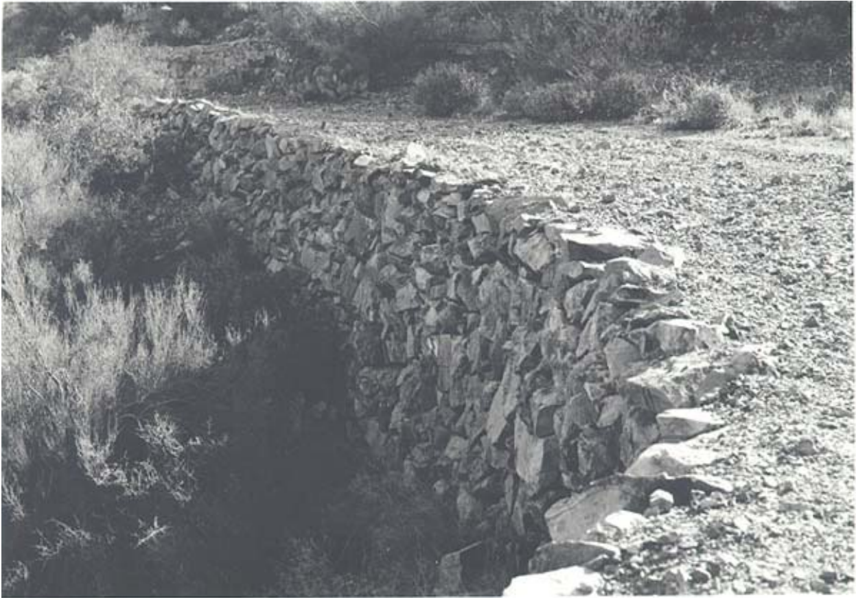
Figure 4. One of the retaining walls built along the King Canyon Road/Trail.
