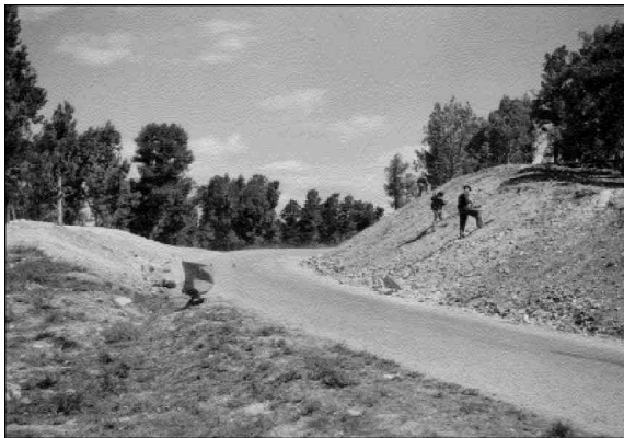
Figure 20.A 1937 Civilian Conservation Corps crew rounding slopes along West Rim Drive. GRCA 281.
