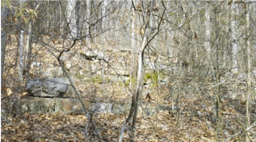
Dry masonry stone foundation belonging to McIntosh livery stable (NPS 2/2005)
