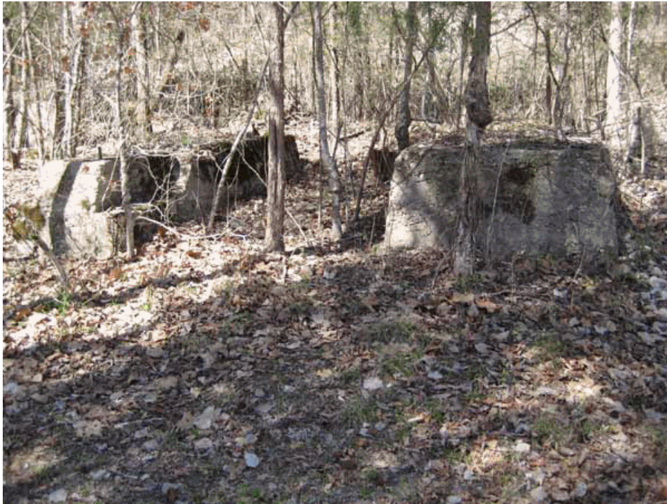
Concrete piers belonging to White Eagle Mill (NPS 3/2011)
