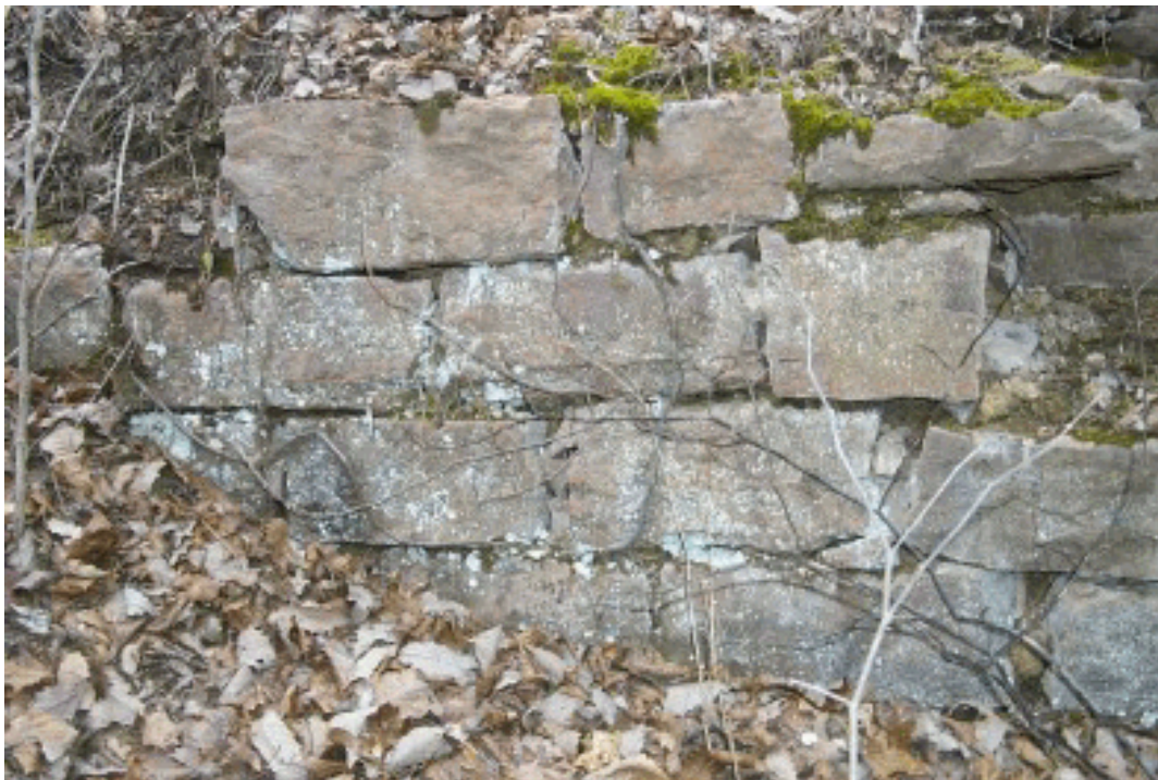
Dry masonry stone wall; component of McIntosh Mill foundation (NPS 2/2005)
