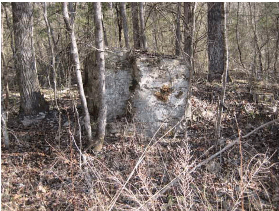
Dry masonry stone wall; component of McIntosh Mill foundation (NPS 2/2005)
