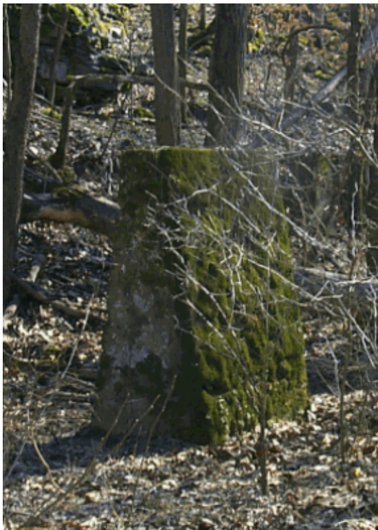
Concrete pier belonging to Red Cloud Processing Mill (NPS 2/2005)
