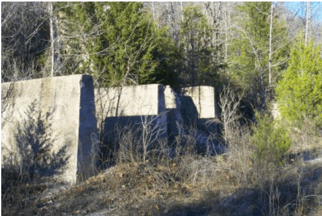
White Eagle Mine New Mill Piers (NPS 12/2004)
