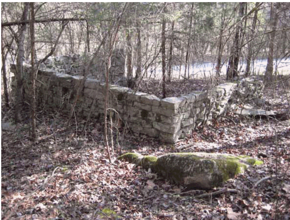
Coursed, mortared stone foundation belonging to the only remaining building in New Town (NPS 3/2011)
