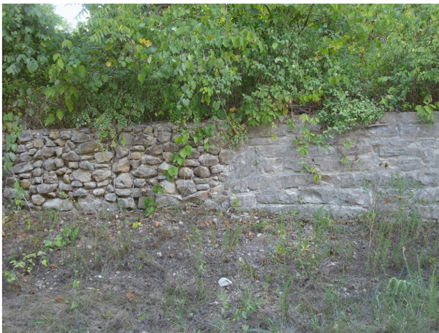
Two masonry campaigns visible on Hicks Wall (Jackson/NPS 2012)
