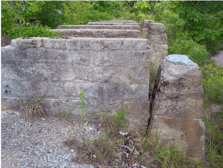
Series of concrete piers belonging to Morning Star Mill (Jackson/NPS 2012)
