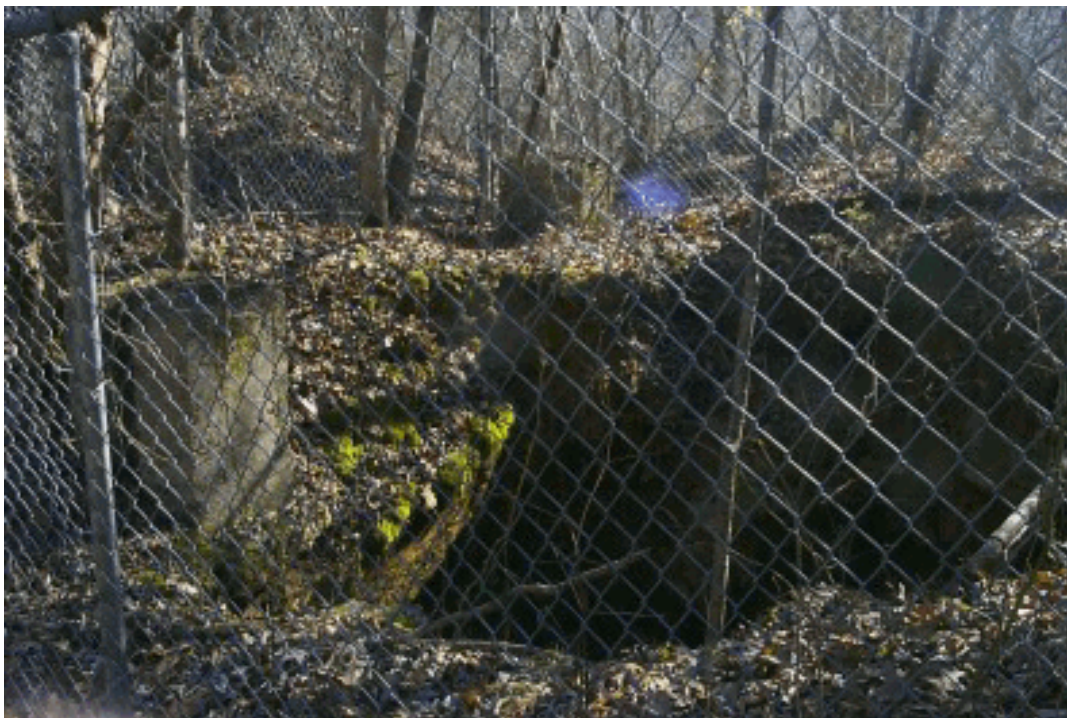
Fenced entrance to Edith Mine shaft (NPS 12/2004)
