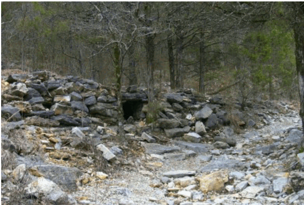
Stone retaining wall and culvert along Morning Star Roadbed (NPS 2/2005)
