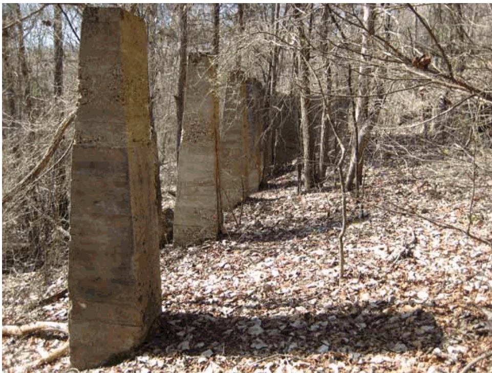
Piers belonging to Edith Mine Processing Mill (NPS 3/2011)
