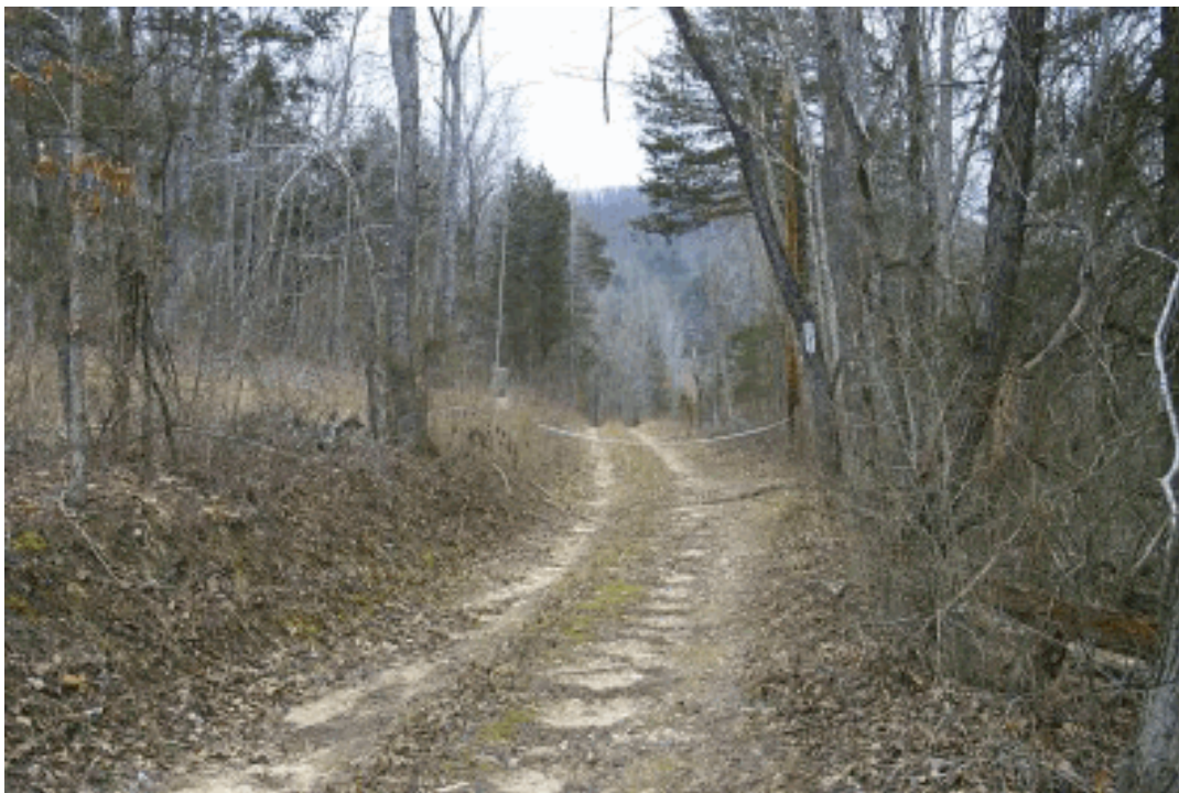
Clabber Creek Roadbed (NPS 2/2005)
