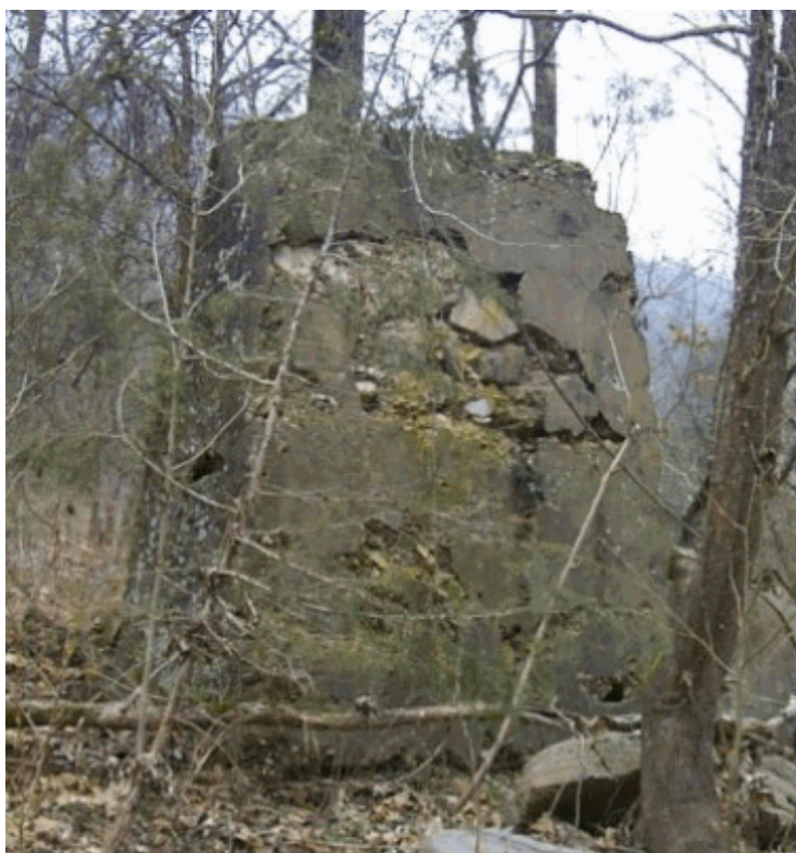
Rubble stone and concrete pillar belonging to footbridge over Rush Creek (NPS 2/2005)
