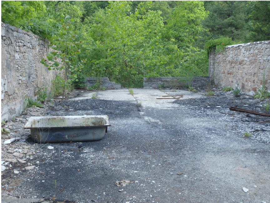
Remaining ashlar walls of Hicks General Store, destroyed by arson in 2004 (Jackson/NPS 2012)
