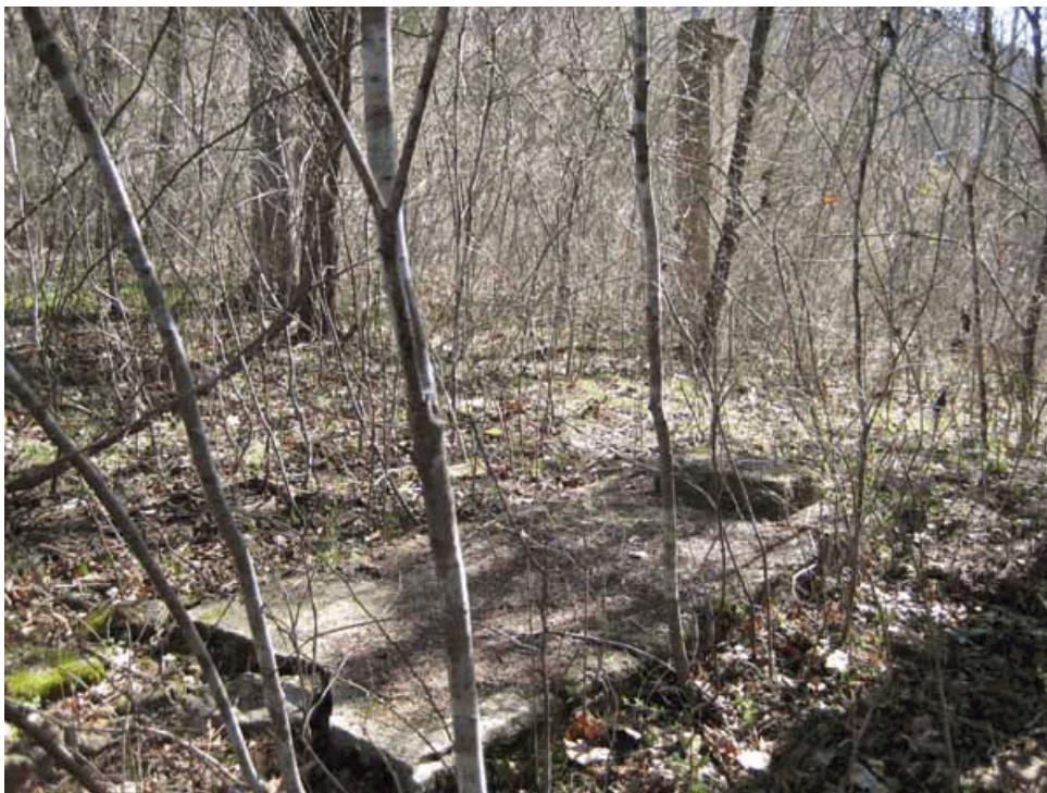
Remnant concrete pad foundation, sidewalk, and brick chimney belonging to manager's house at Morning Star Mill (NPS 3/2011)
