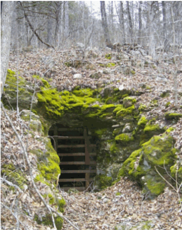
Gated entrance to McIntosh Mine (NPS 2/2005)
