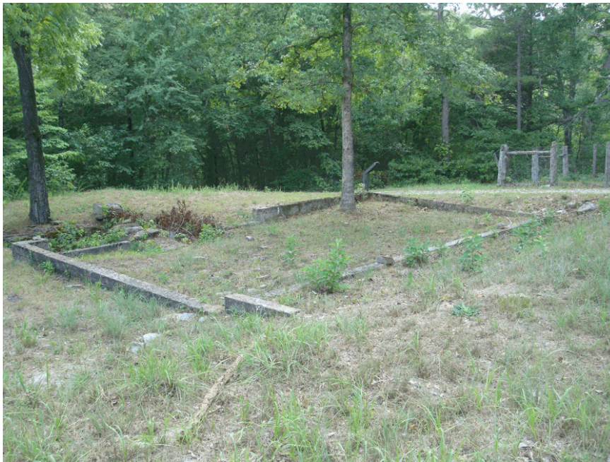
Foundation ruin to the Chase & Mulholland Store (Jackson/NPS 2012)
