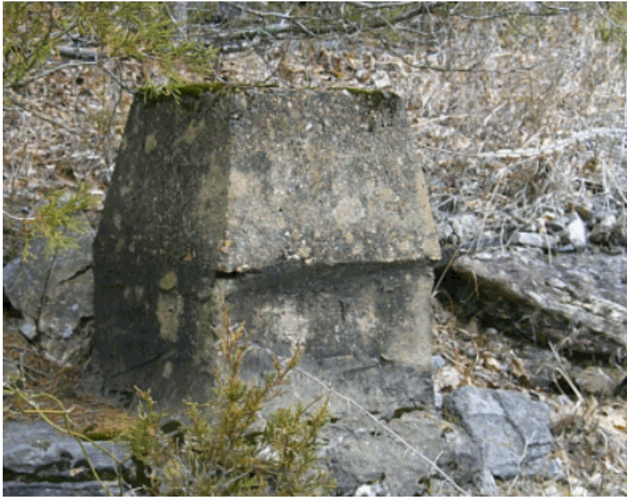
Morning Star Mining Company tramway pier (NPS 2/2005)
