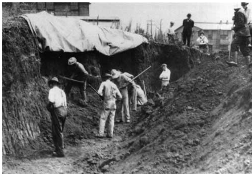
Figure 12: Excavation of Mound 7. (NPS/1920-21)
