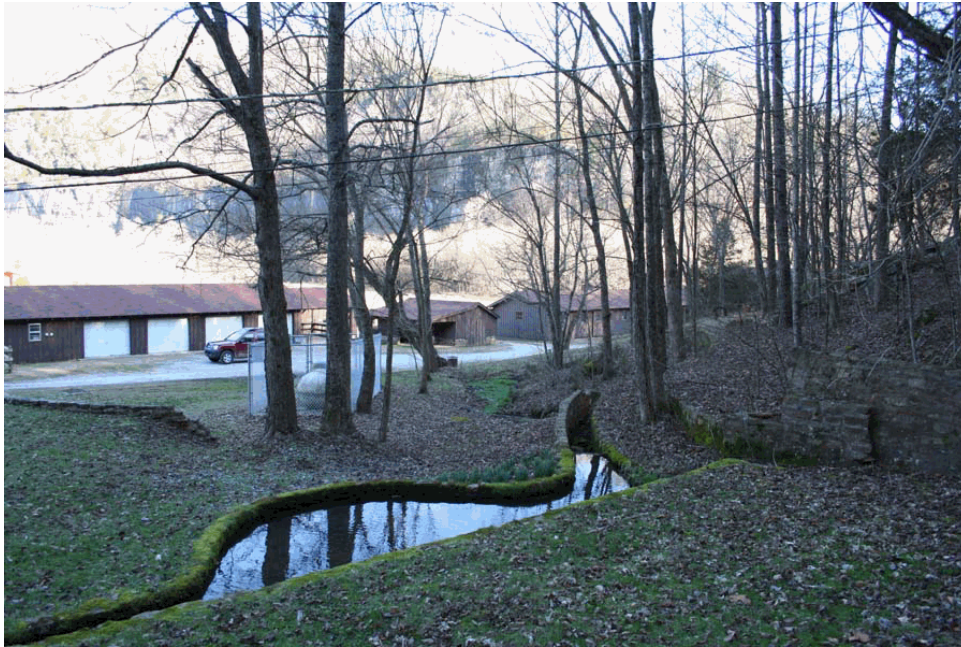
Pond located below the well as it drains into the culvert portion of the system (NPS, 2007).
