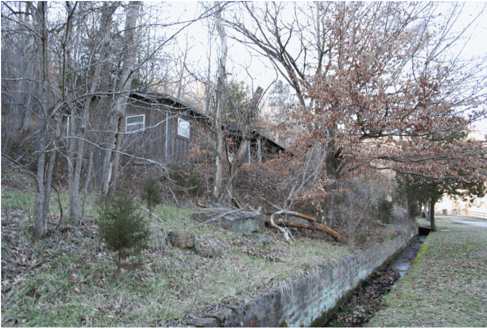
Stone-lined culvert near the Manager's House looking back towards the Rock House (NPS, 2007).
