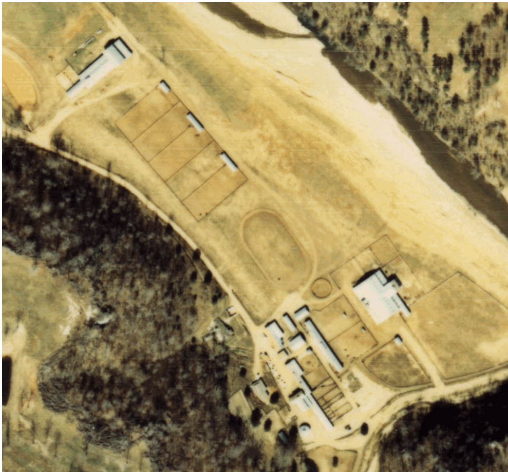
Aerial photo of the ranch dated 1972 shows all the structures and their organization with the valley (NPS archives).
