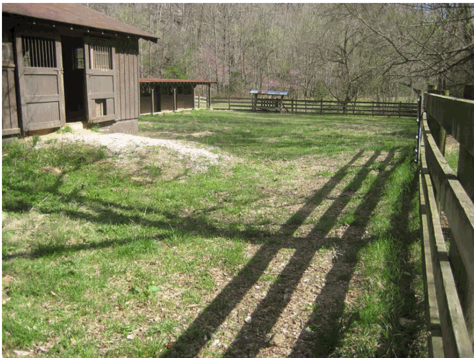
Current fencing located behind the Main Stable (NPS, 2009).
