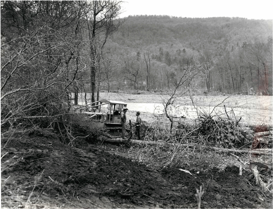
Clearing along the Buffalo River (Yarborough family archives, 1969).
