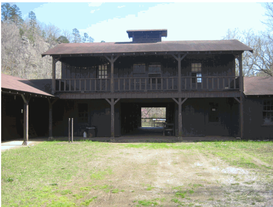
Two-story section of the Main Stable (NPS, 2009)
