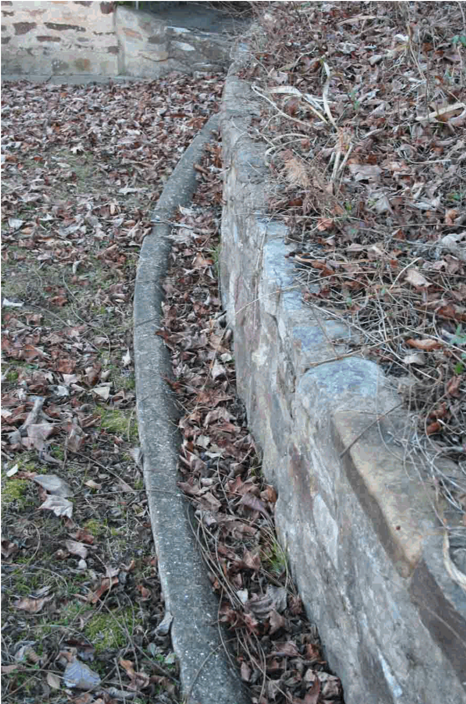
Concrete gutter found around the Rock House (NPS, 2009).
