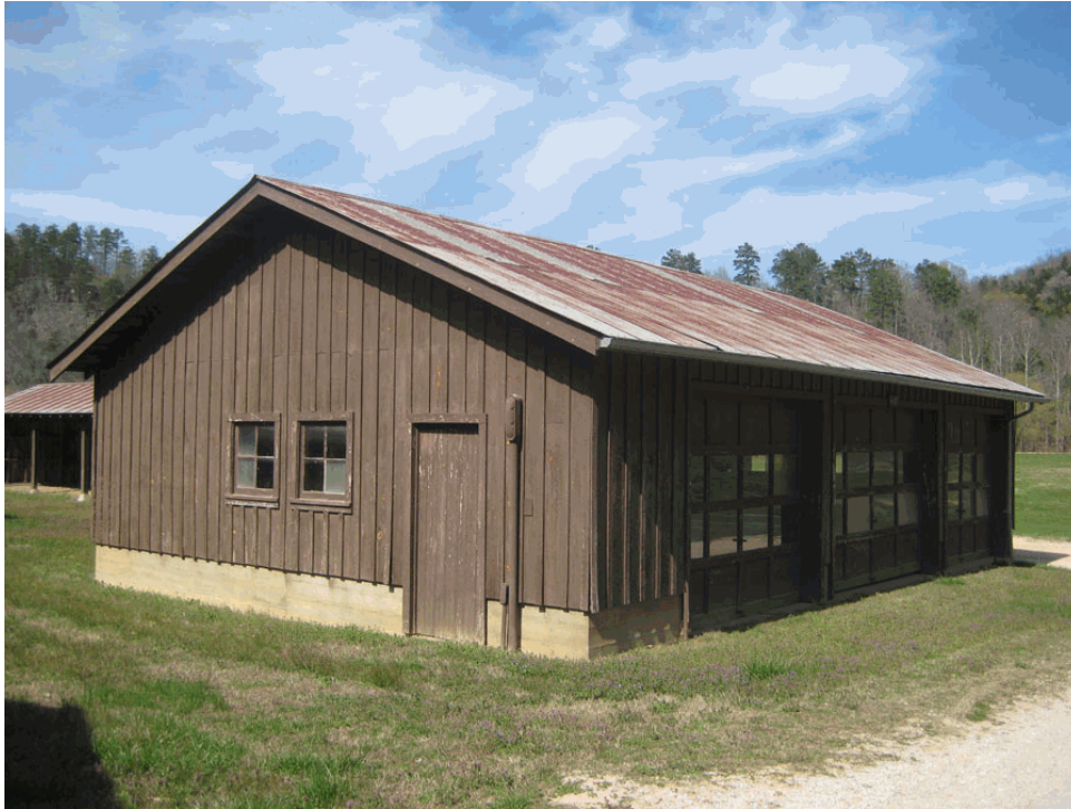
The Machine Shed (NPS, 2009).
