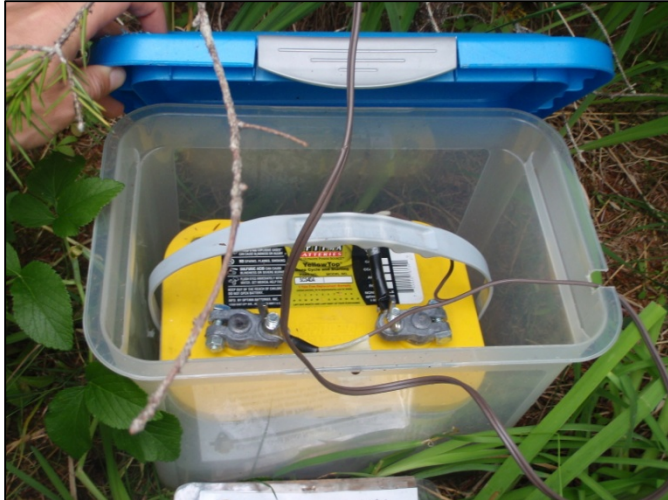
Figure17. Gel cell battery in housing.
