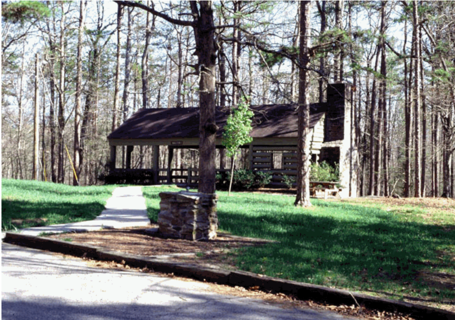
Fig. 15. Photo of CCC Structure in Kings Mountain State Park.
