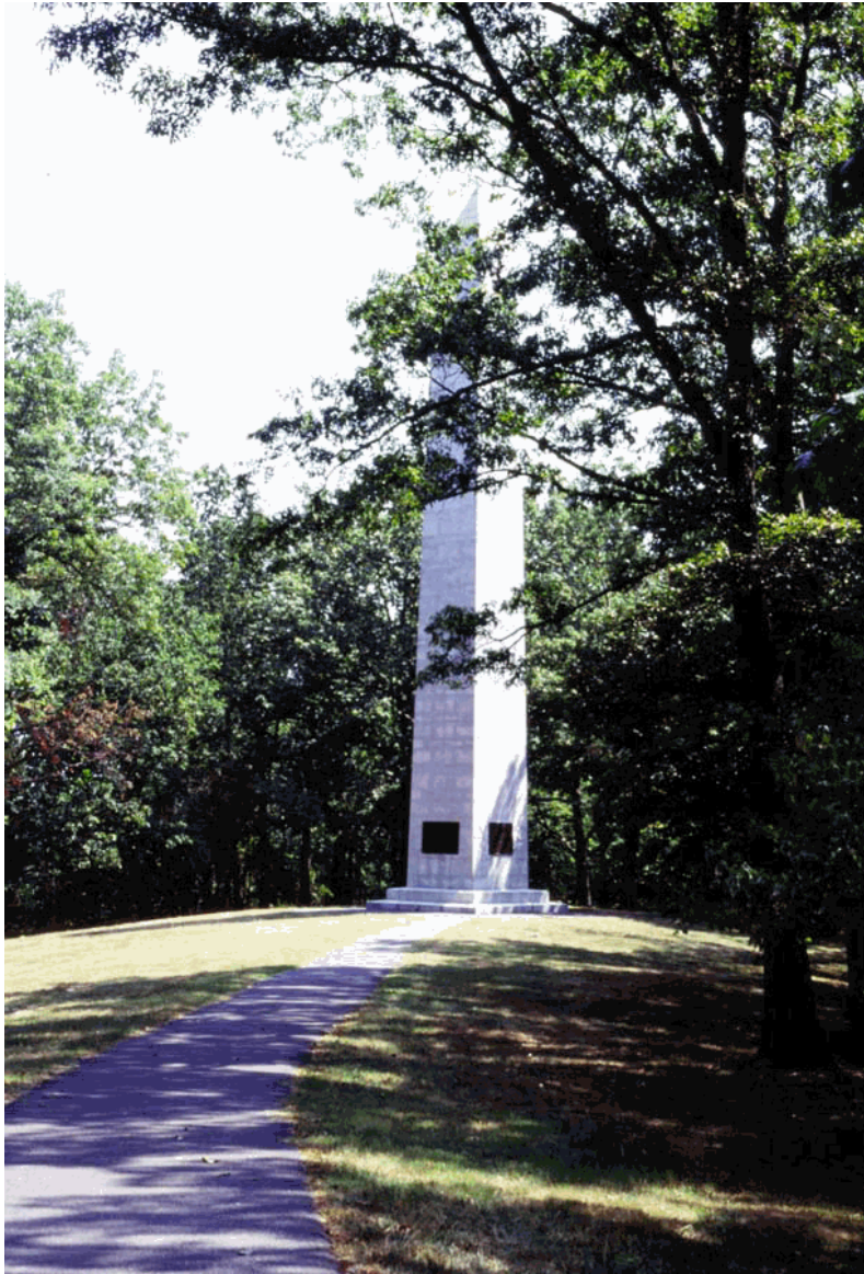
Fig. 12. U.S. Monument, constructed in 1909.
