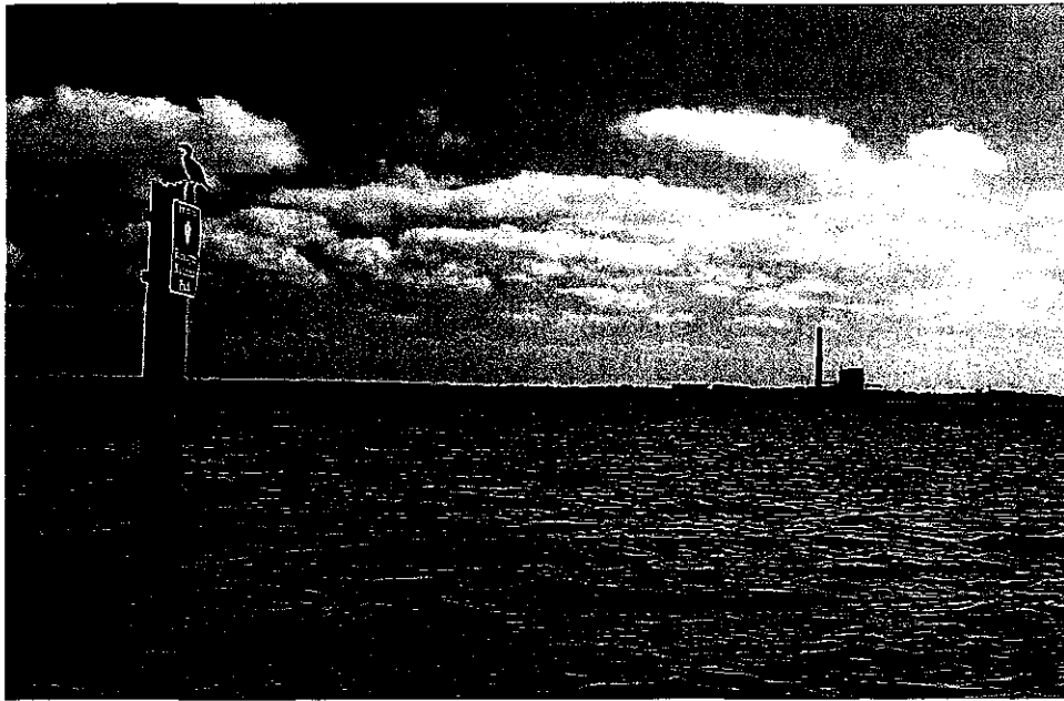
Turkey Point Nuclear Power Plant from vantage point of channel near Convey Point
