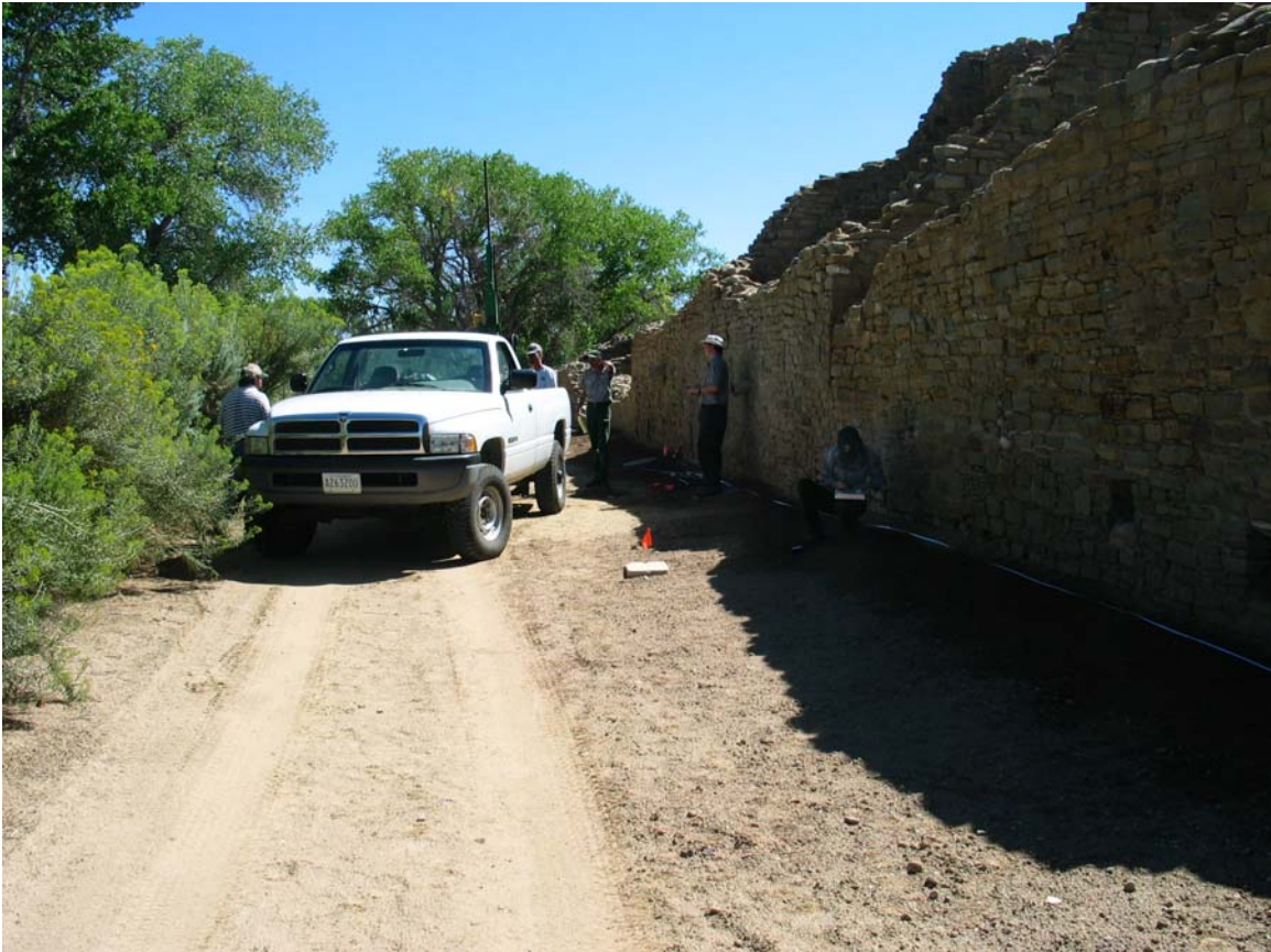
Photograph 1. Installation of hydrologic monitoring instrumentation (August 2005).
