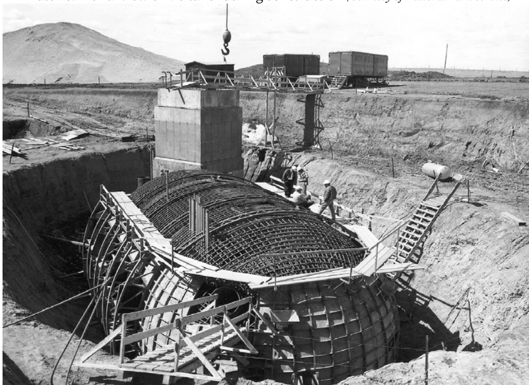
Plate 29. Launch Control Center under construction in South Dakota (Courtesy of Peter Kiewit and Sons', Inc.)
