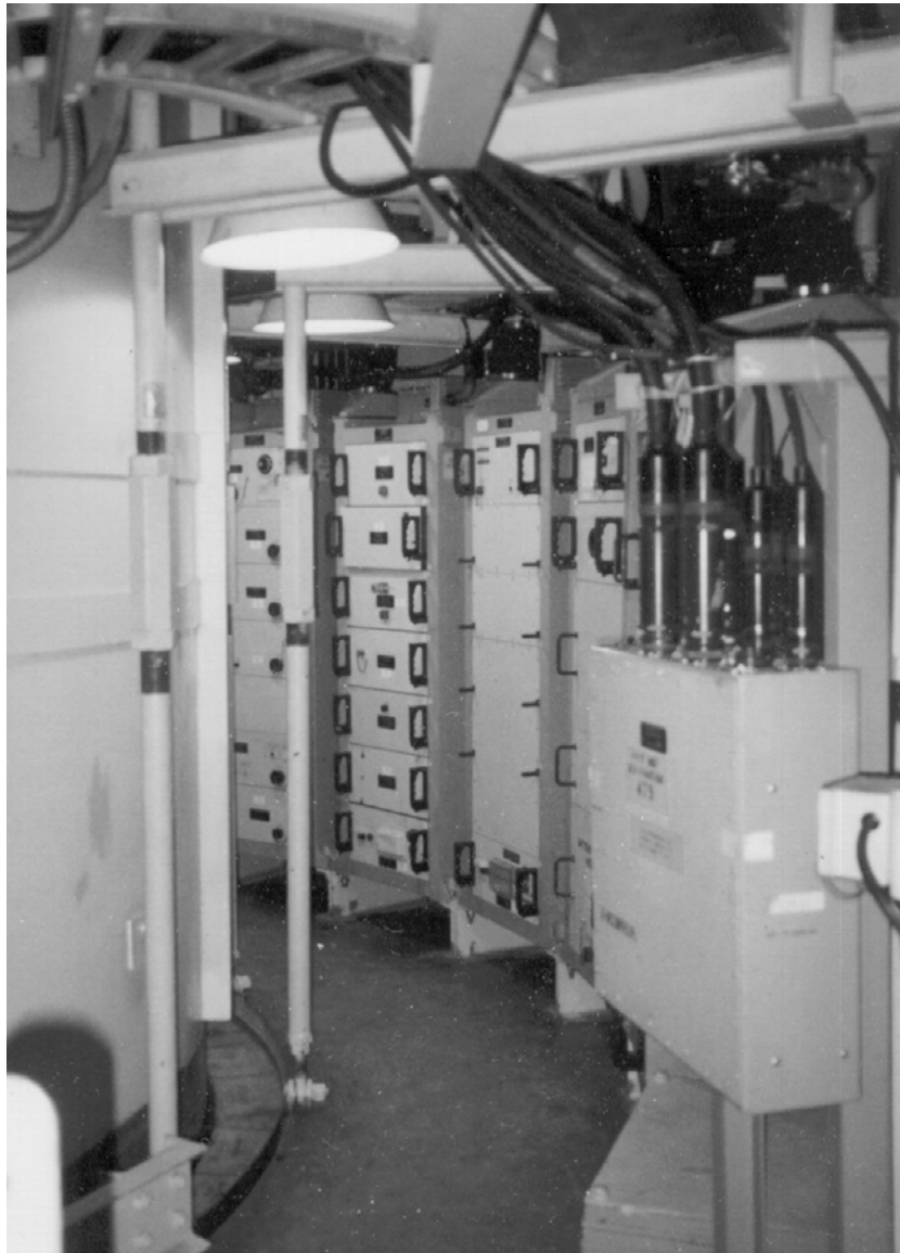
Plate 53. Interior of Delta-09 silo showing launch tube encircled by electronic equipment (Courtesy of National Park Service, Photograph by Richard M. Kohen)
