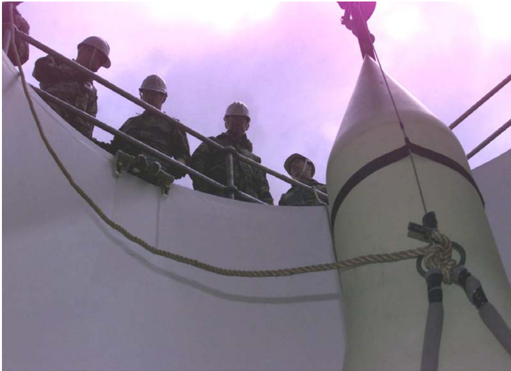
Plate 84. Training missile emplacing, Delta-09 silo (Photograph by Staff Sergeant Melissa Phillips, F.E. Warren Air Force Base, Wyoming, U.S. Air Force photo)
