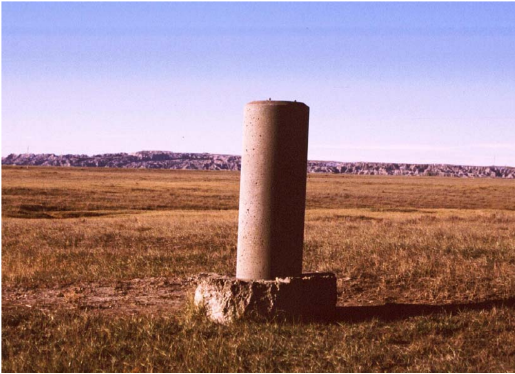
Plate 54. One of two azimuth markers located outside the Delta-09 security fence used by guidance technicians to align the missile's guidance system ( Photograph by Mead & Hunt, Inc. )
