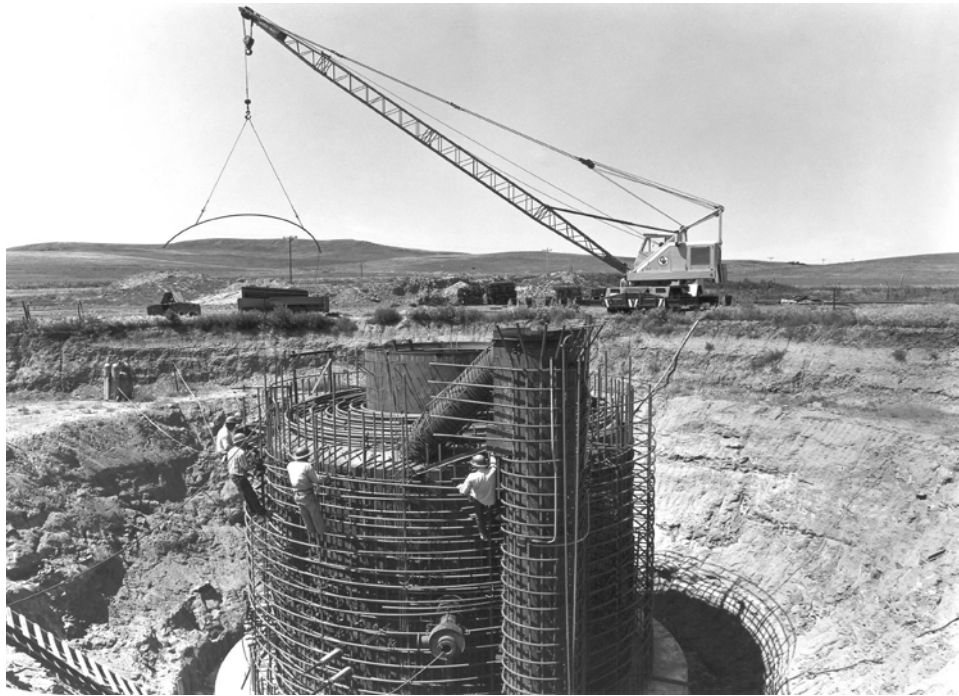
Plate 32. Launch tube under construction in South Dakota ( Courtesy of Peter Kiewit and Sons', Inc. )
