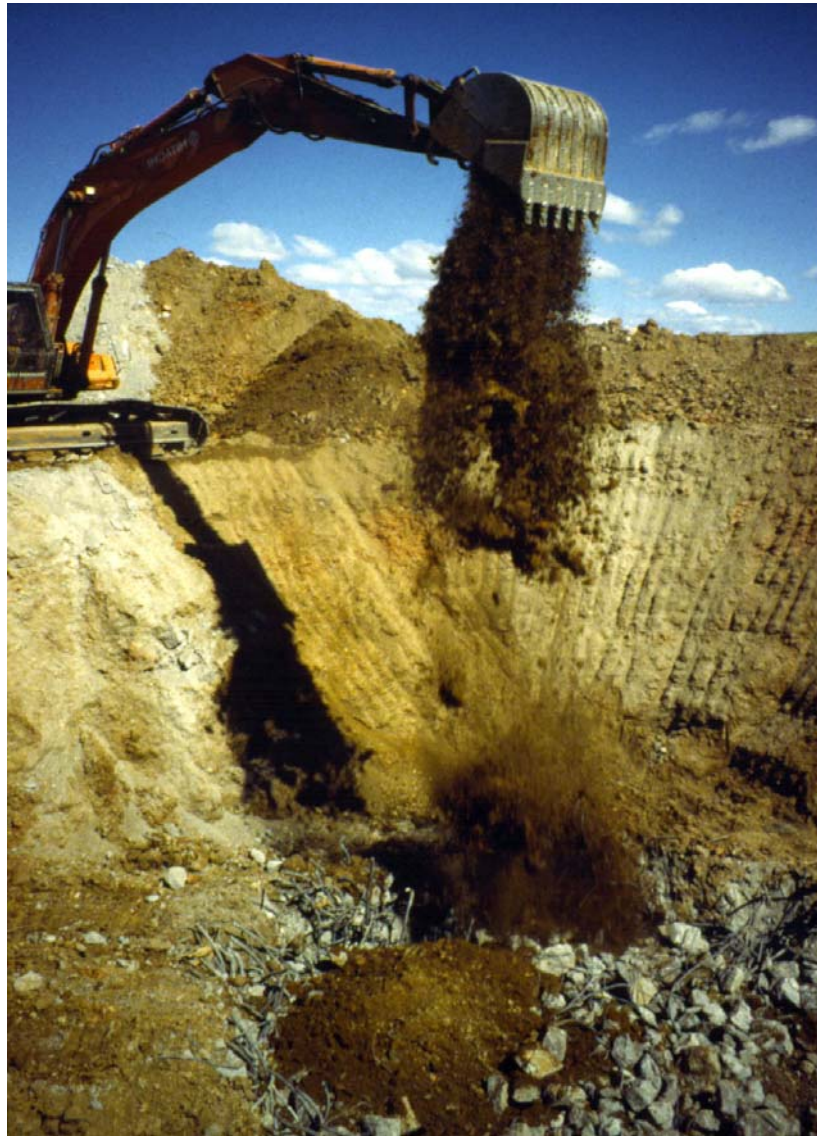
Plate 79. Missile silo being filled after implosion, South Dakota (Courtesy of the 28 th Civil Engineer Squadron, Ellsworth Air Force Base)
