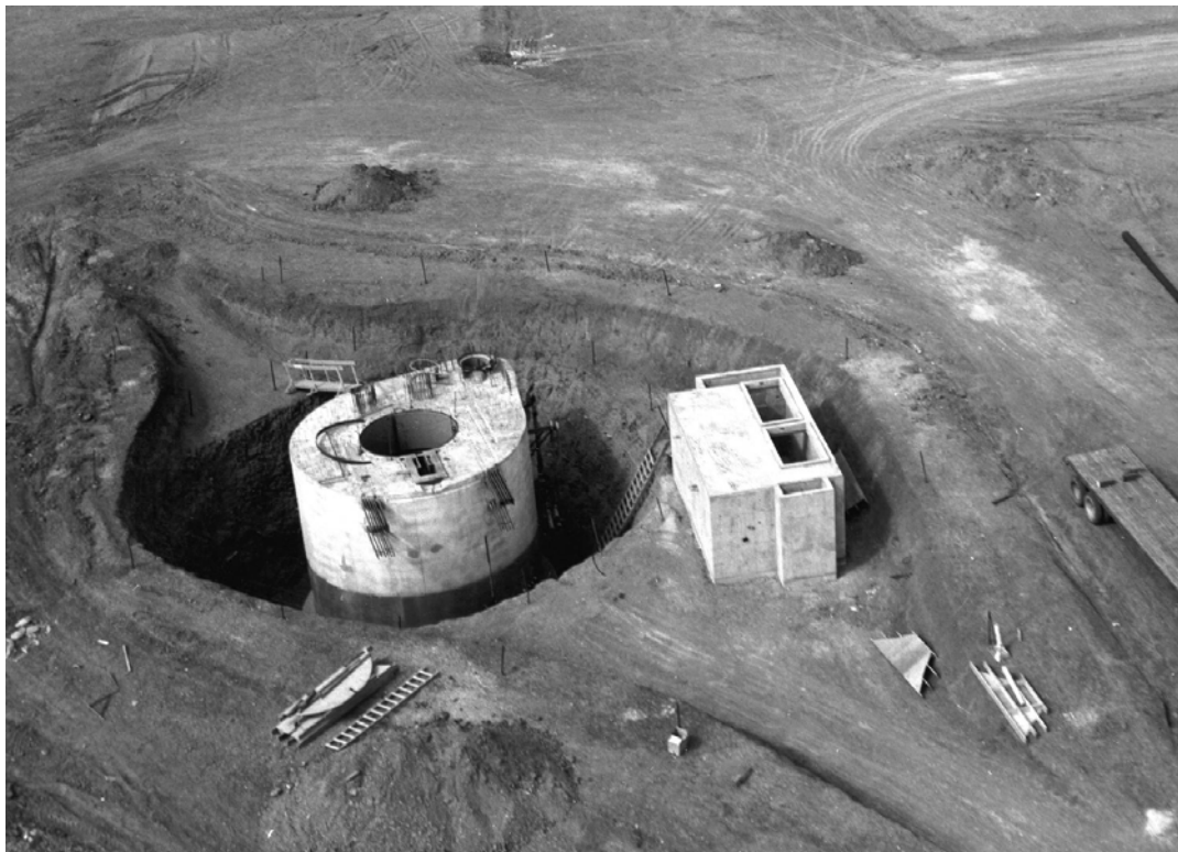
Plate 33. Aerial view of a launch tube under construction in South Dakota ( Courtesy of Peter Kiewit and Sons', Inc. )
