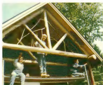
Young volunteers help "top off" a new ranger station at Malone Bay.
