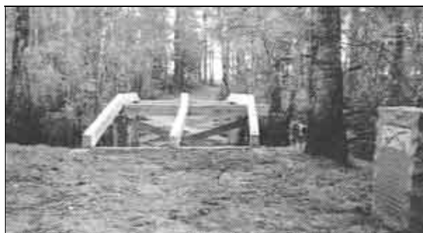
Figure 14. The completed bridge reconstruction, 1992.
