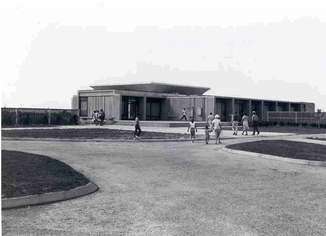
Approach to visitor center showing cypress fence, 1960
