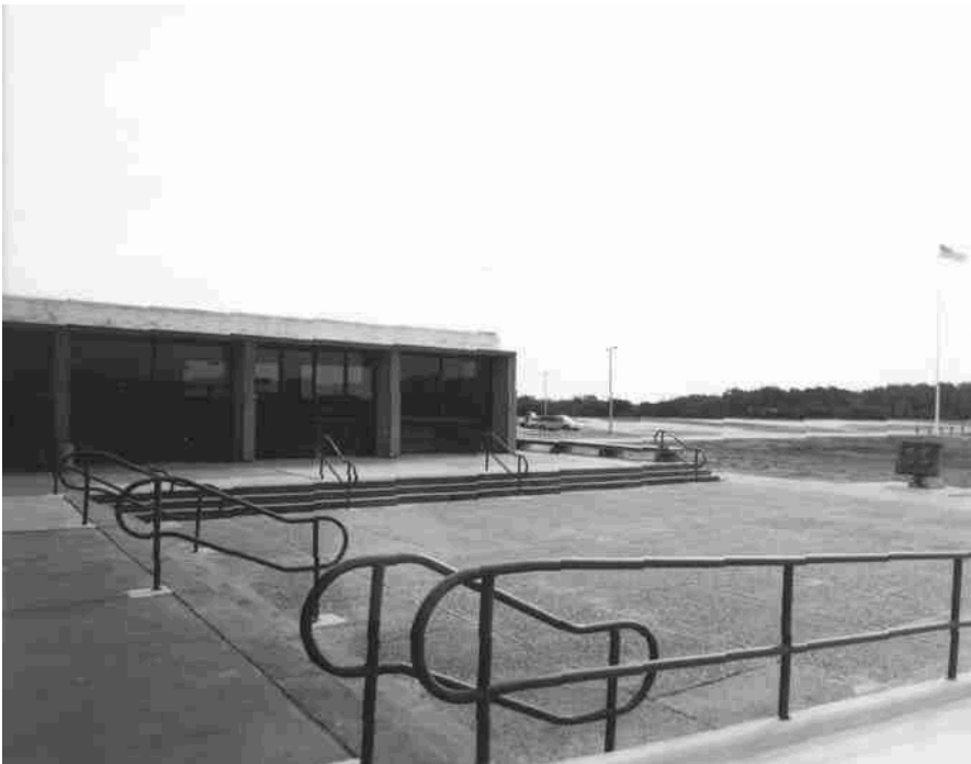
Handicapped rails and concrete repairs, 2000
