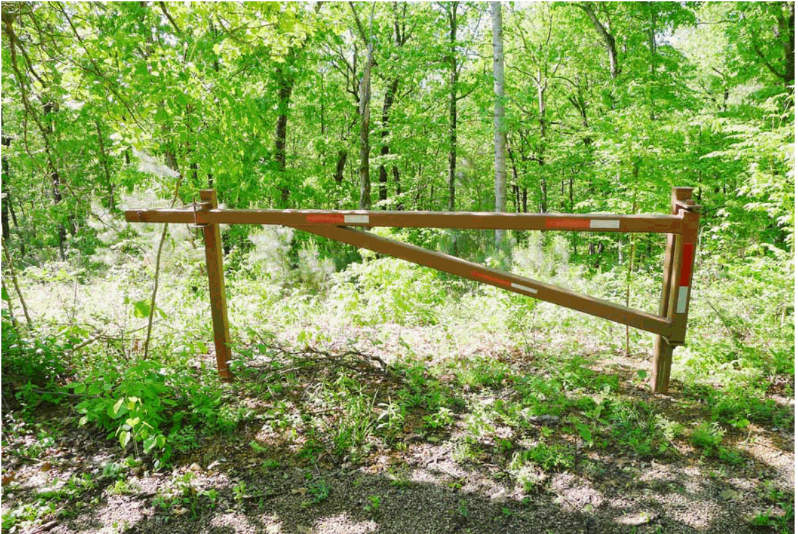
Modern NPS steel gate at Fort Heiman, 2010. TJC Photo.
