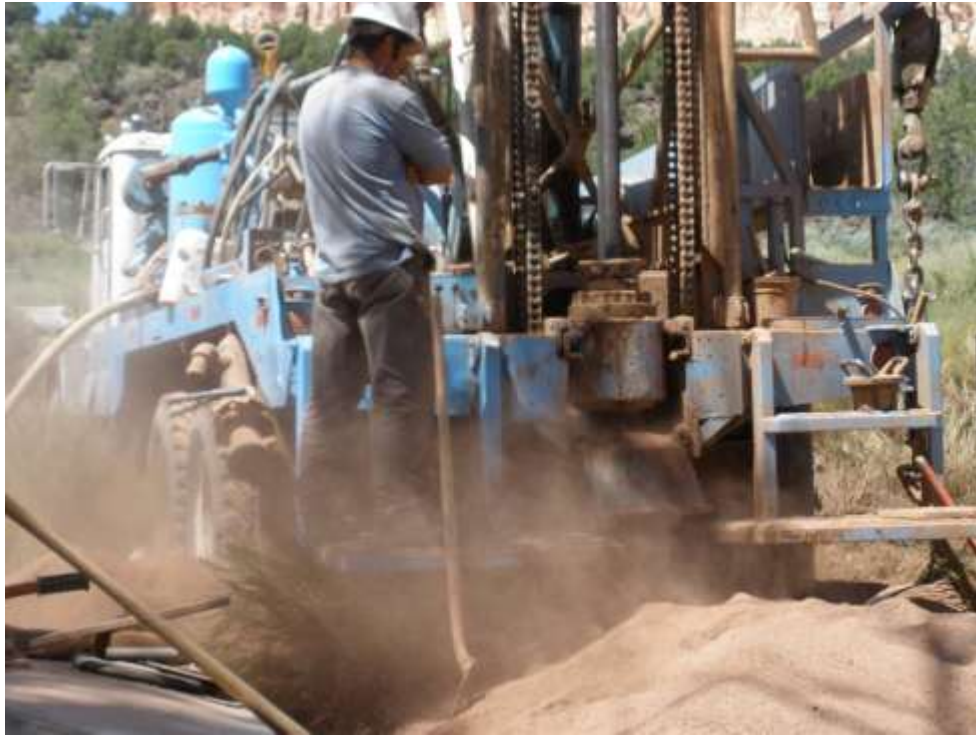
Photo during drilling of the test hole. The dry dust provides evidence of the lack of water.
