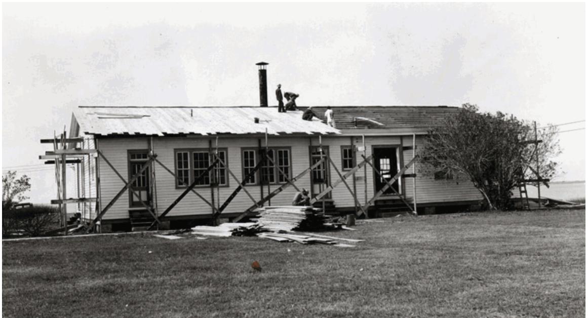
Figure 49. Frame utility building, 1940. Fort Pulaski National Monument archives
