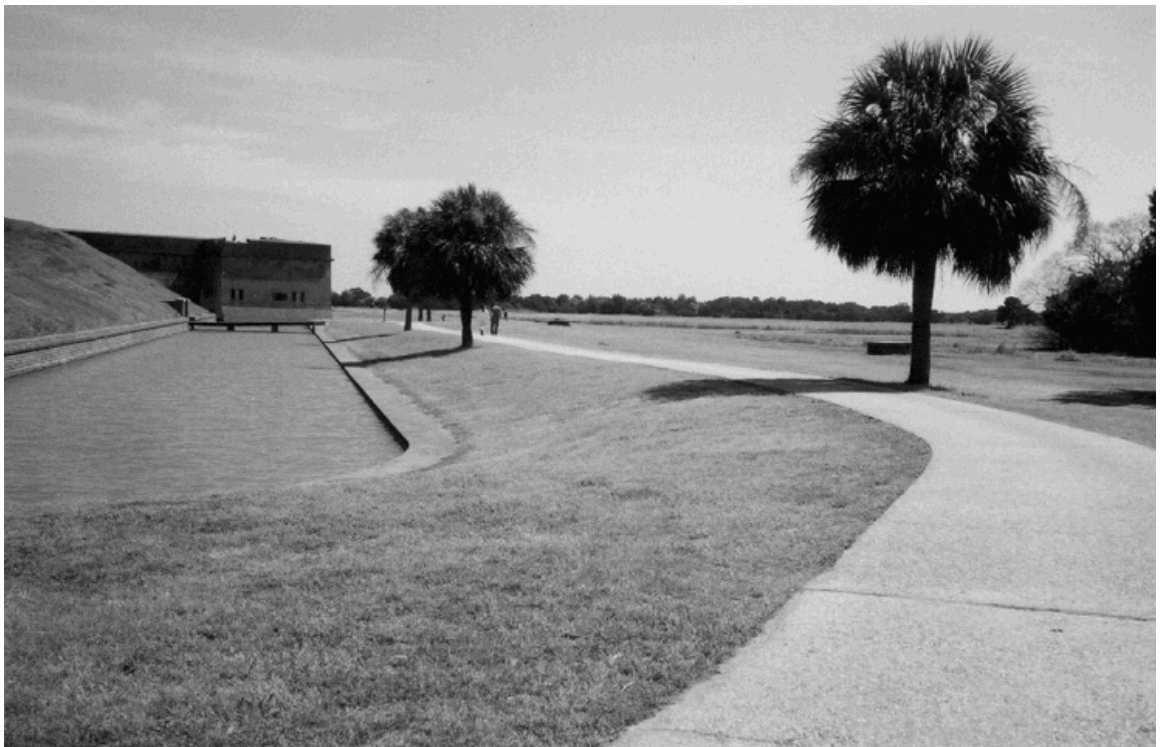
Figure 62. Exposed Aggregate Walkway, 2005. NPS photo (walktofortdemilune)
