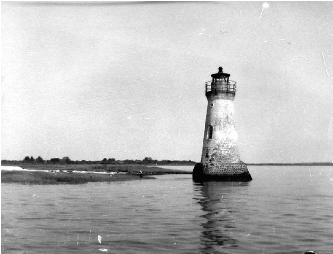
Figure 24. Cockspur Island Lighthouse, 1950's. Fort Pulaski National Monument archives
