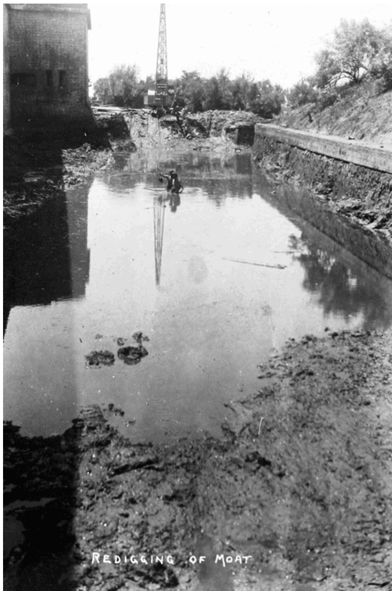
Figure 18. Moat excavation by CCC workers. Fort Pulaski National Monument archives
