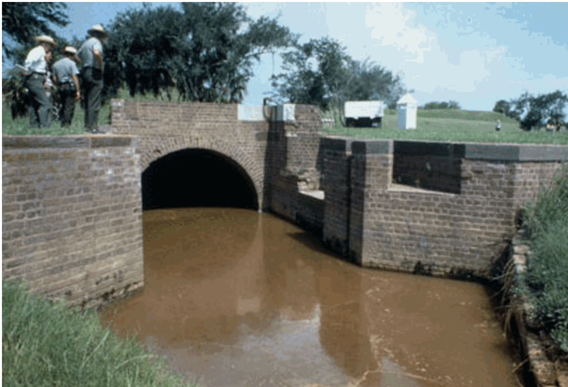
Figure 71. Canal Lock. NPS photo
