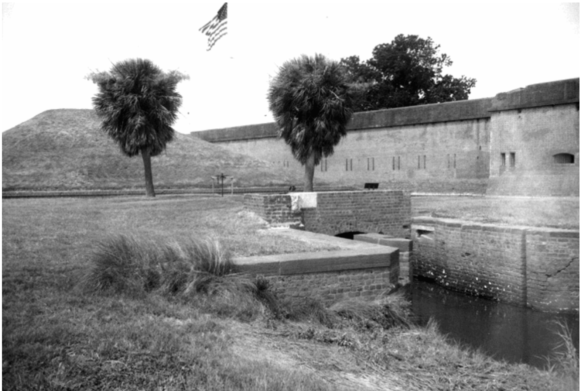
Figure 68. North Tide Gate, 2007. NPS Photo.
