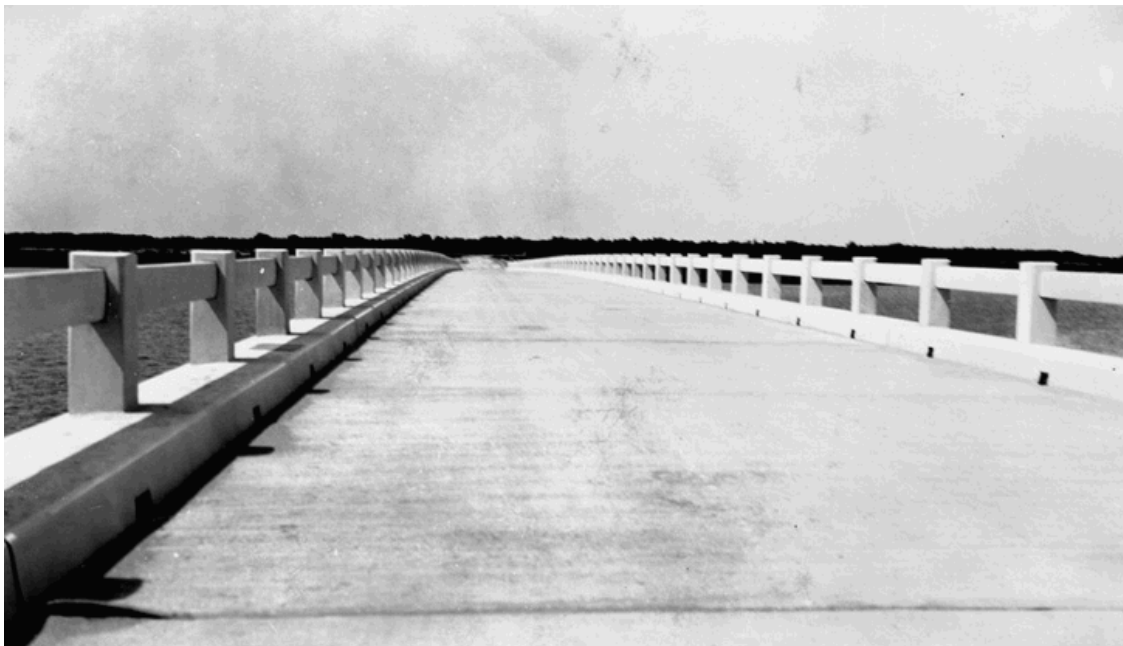
Figure 19. South Channel Bridge, 1938. Fort Pulaski National Monument archives
