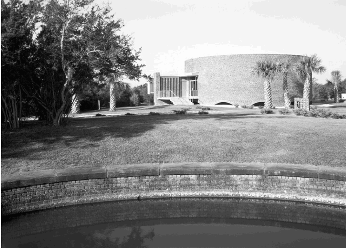
Figure 21. Fort Pulaski visitor center. Jack E. Boucher/NPS
