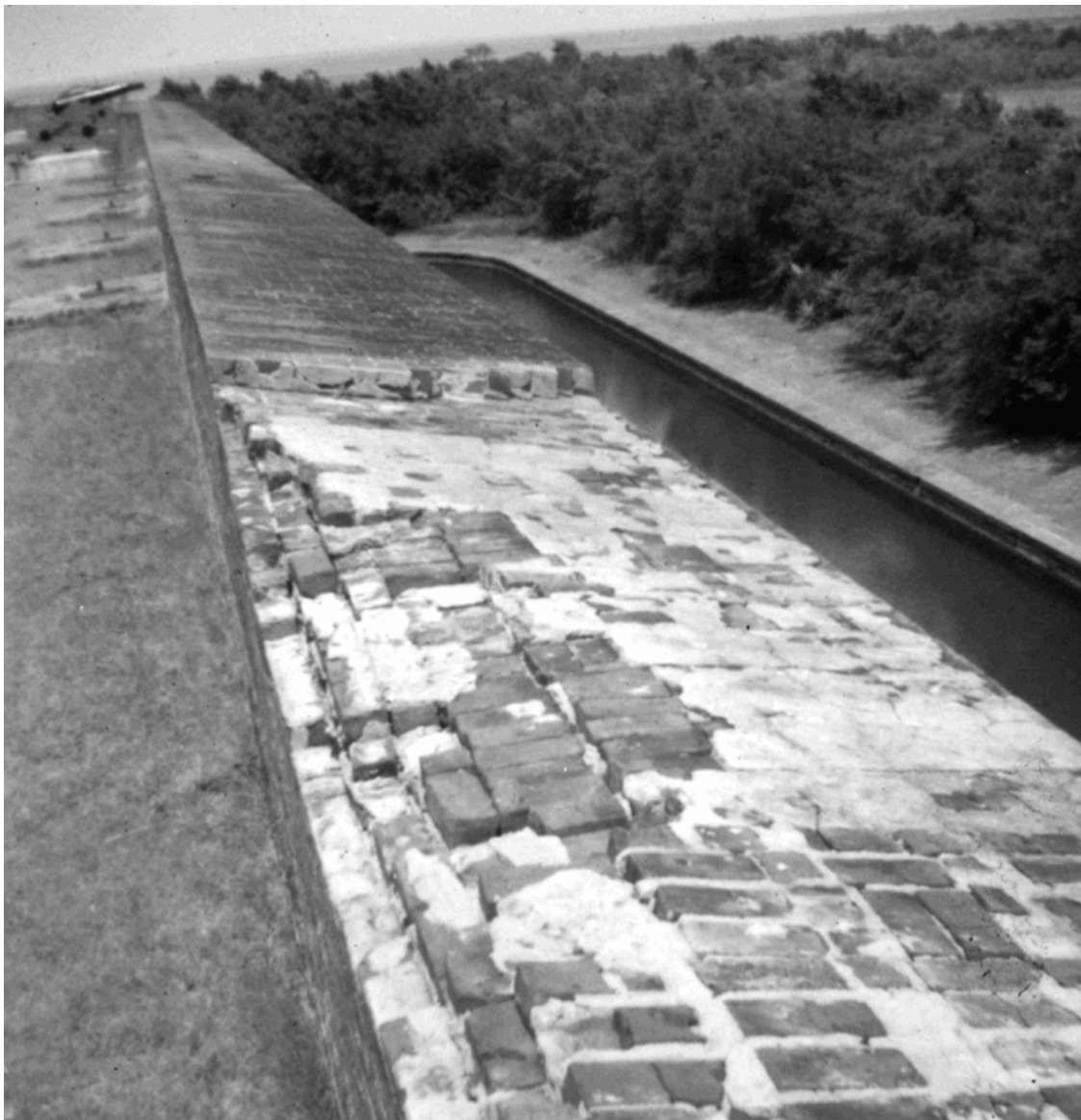
Figure 22. Parapet before repairs in 1958. NPS image
