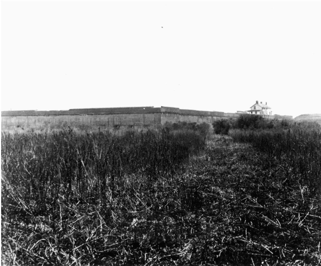
Figure 17. Lightkeeper's house on terreplein. FOPU Archives
