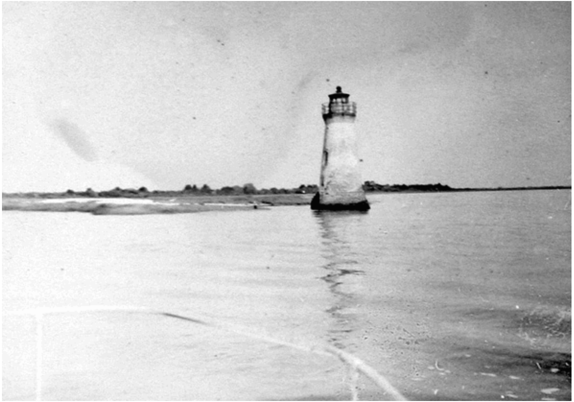
Figure 39. Cockspur Island Lighthouse, 1950s. Fort Pulaski National Monument archives
