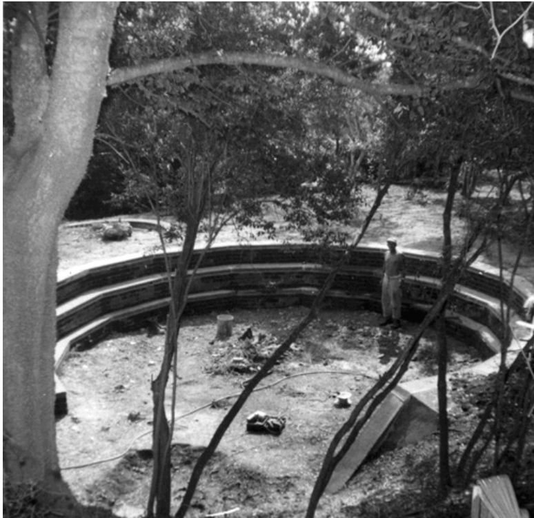
Figure 32. Repair work to pintle gun pit, c.1936. Fort Pulaski National Monument archives
