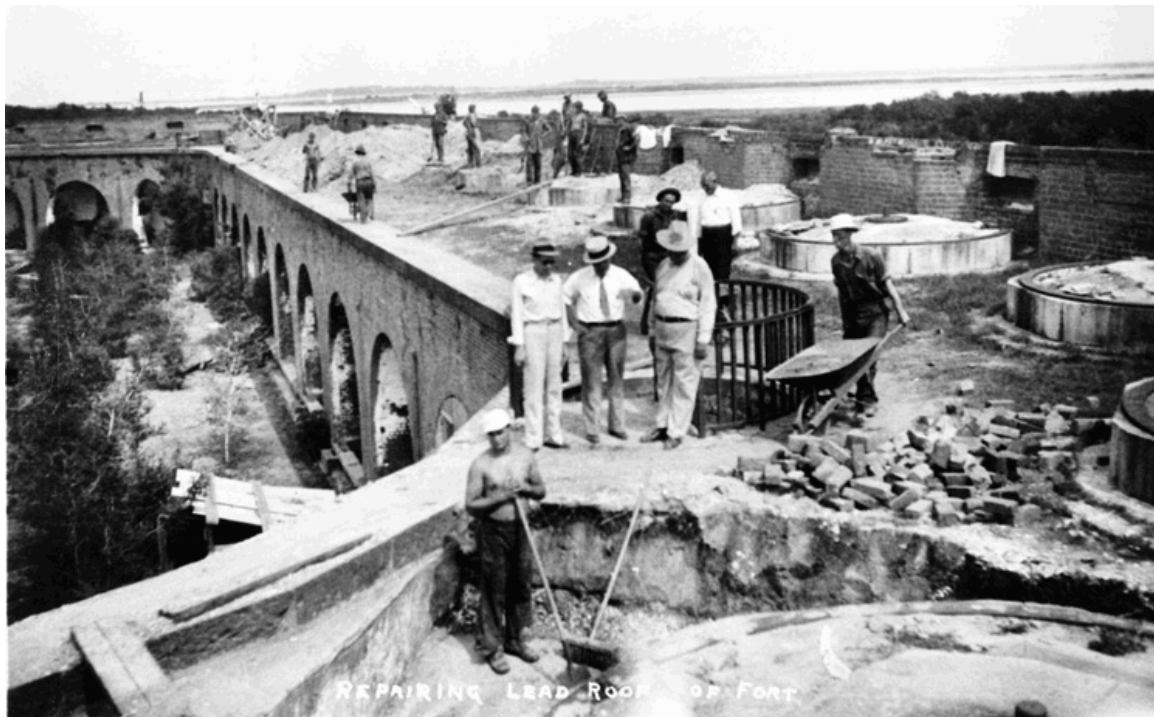
Figure 30. Lead roof repair, n.d. Fort Pulaski National Monument archives
