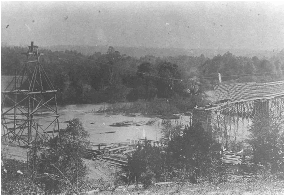
Construction of Miller covered bridge, 1907-1908.
