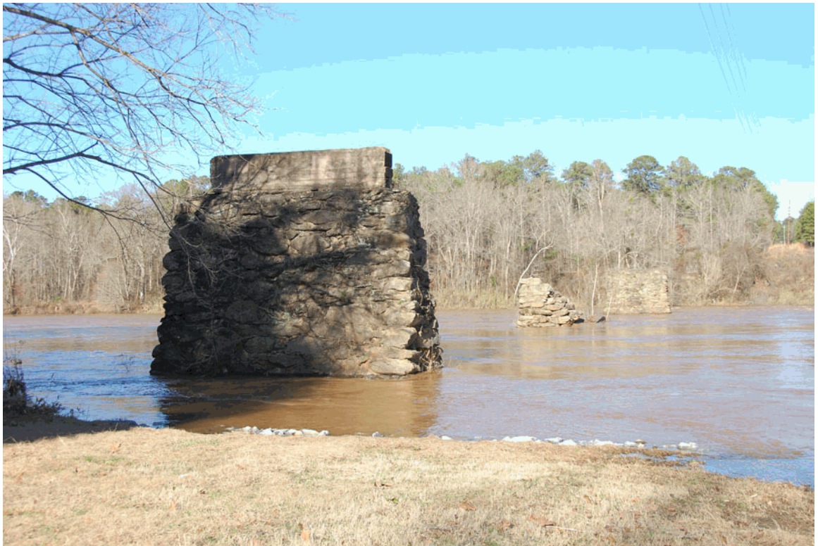
Miller Bridge piers, 2012.
