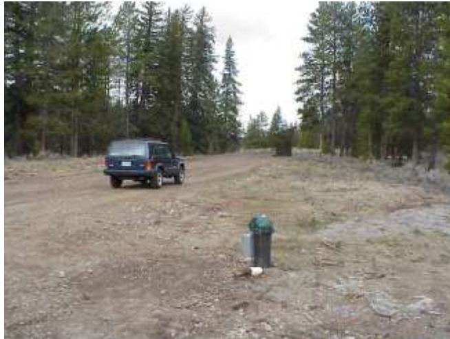
View of the new well at Moran Junction. View is toward the North. Snake River is behind the trees on the left side of the photo.
