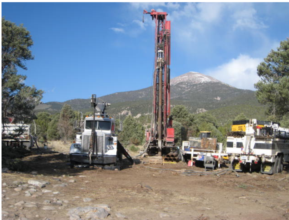
Figure 3. Photograph of well site 1 east of sewage lagoons at Great Basin National Park, White Pine County, Nevada showing drill rig, 20-ft length of nominal 10-inch casing attached to top driver hammer and diverter with hose to cyclone in dump truck. Also shown are the crane truck, pipe trailer, water truck, and extra air compressor on trailer behind water truck. Photograph was taken May 11, 2012 looking west with Jeff Davis Peak in background.
