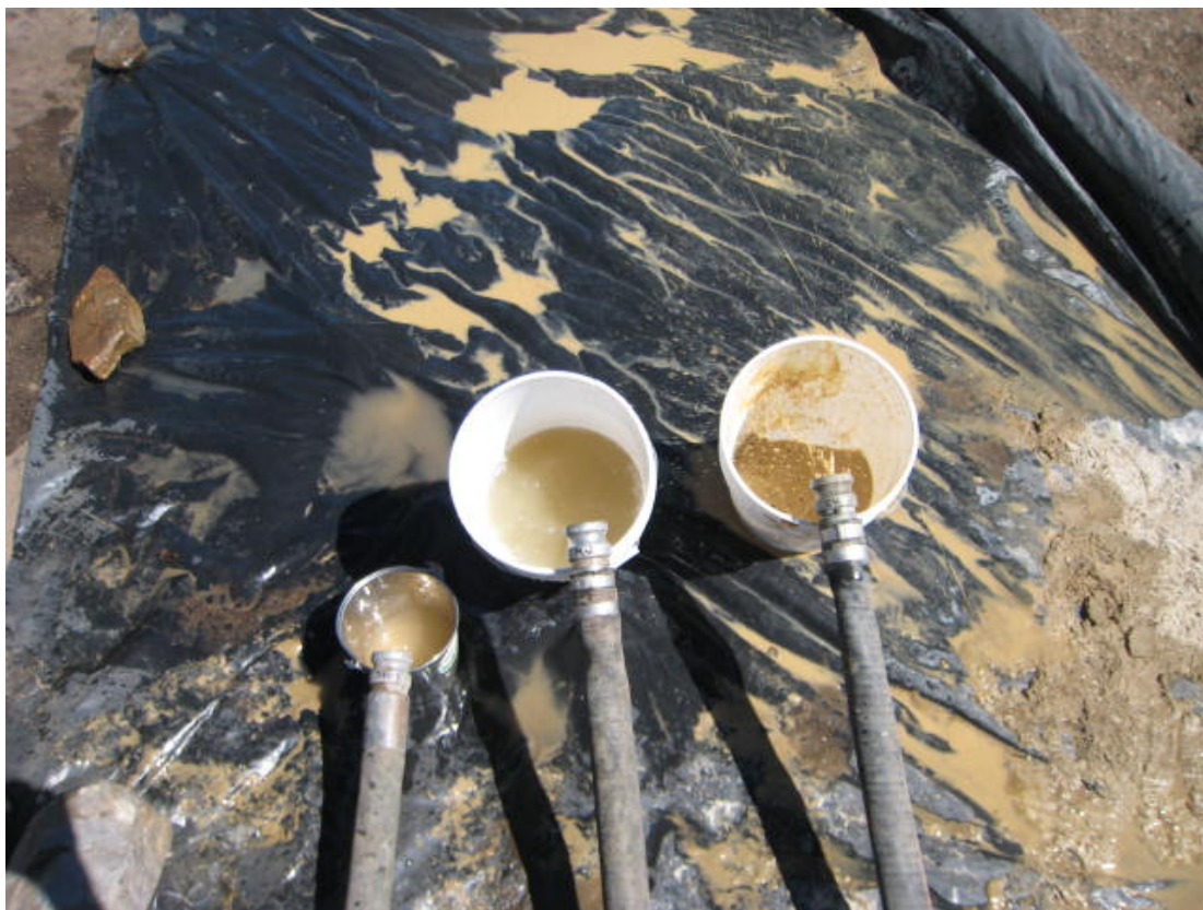
Figure 10. Photograph of water being air lifted out of each well during development at well site 1 east of sewage lagoons, Great Basin National Park, White Pine County, Nevada.
