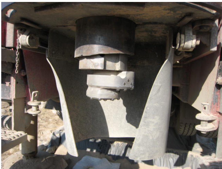
Figure 5. Photograph of new nominal 10-inch shoe with new under-reaming bit extending beyond shoe prior to drilling through the neat-cement-filled hole on May 13, 2012 at well site 1 east of sewage lagoons, Great Basin National Park, White Pine County, Nevada.
