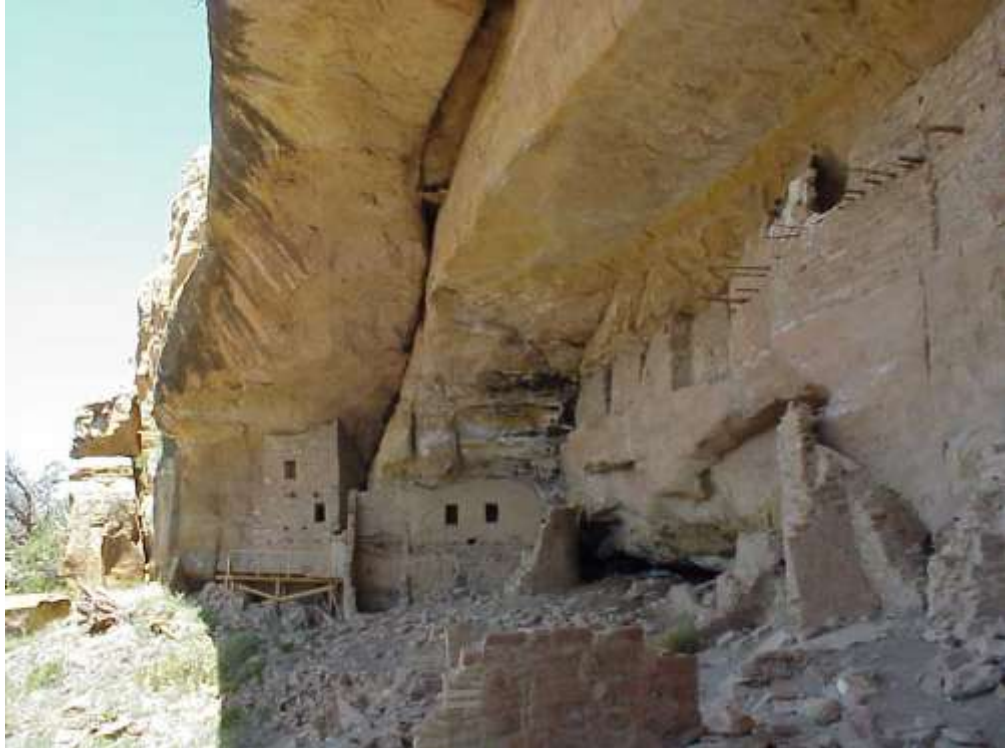
Photo of the northern part of Spring House. The spring is at the intersection of the vertical crack and the base of the cliff, behind the wall in the center of the photo.
