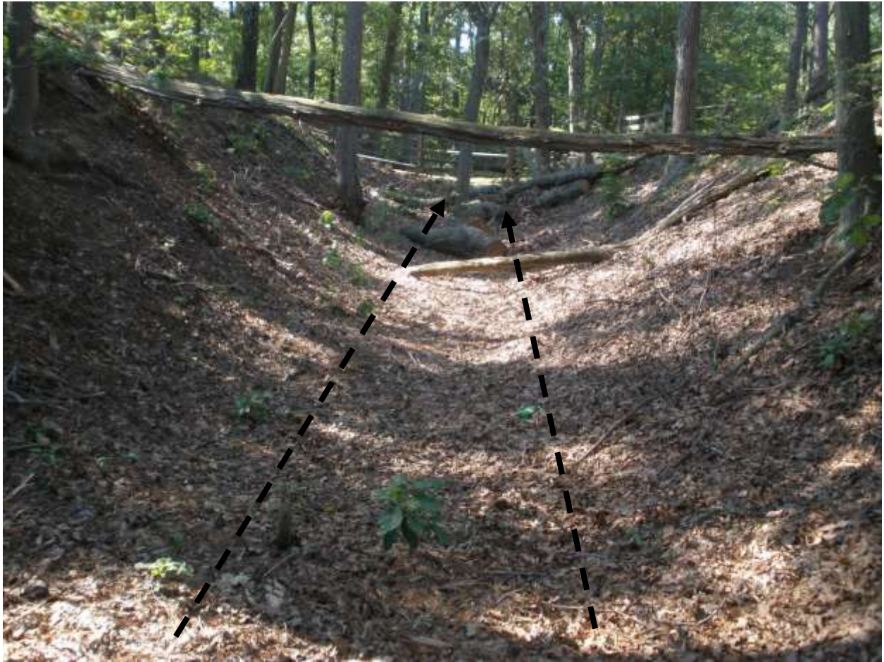
Photo of one of the trenches excavated during the construction of the fort. In this area, two parallel trenches might be constructed with perforated pipe to intercept infiltration and drain the water away from the bluff. Dashed lines show approximate layout of drainage pipe.
