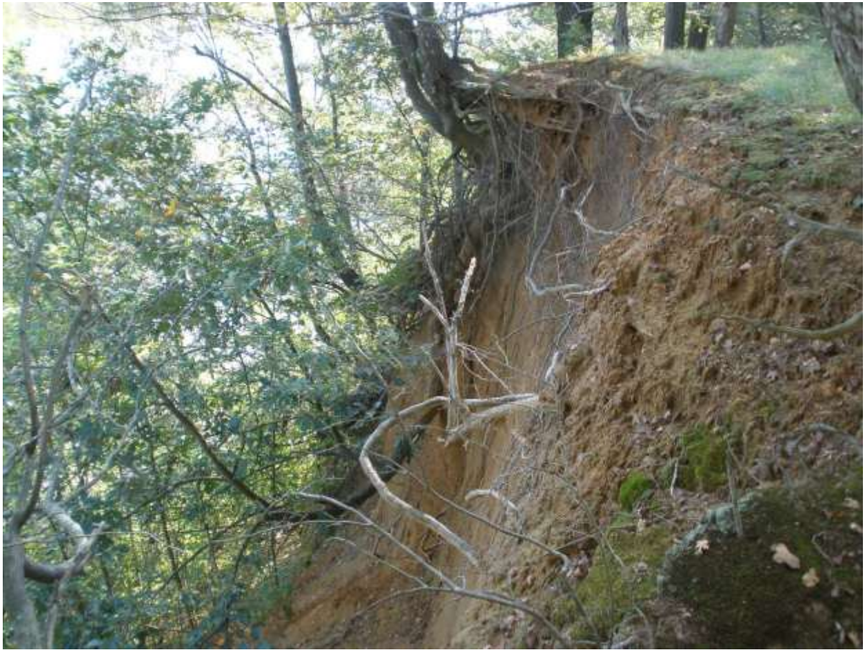
Photo of a near-vertical slope at the top of the bluff. This area is inherently unstable. Slope failure and slumping is inevitable. The material exposed on the bluff face is sand and gravel.
