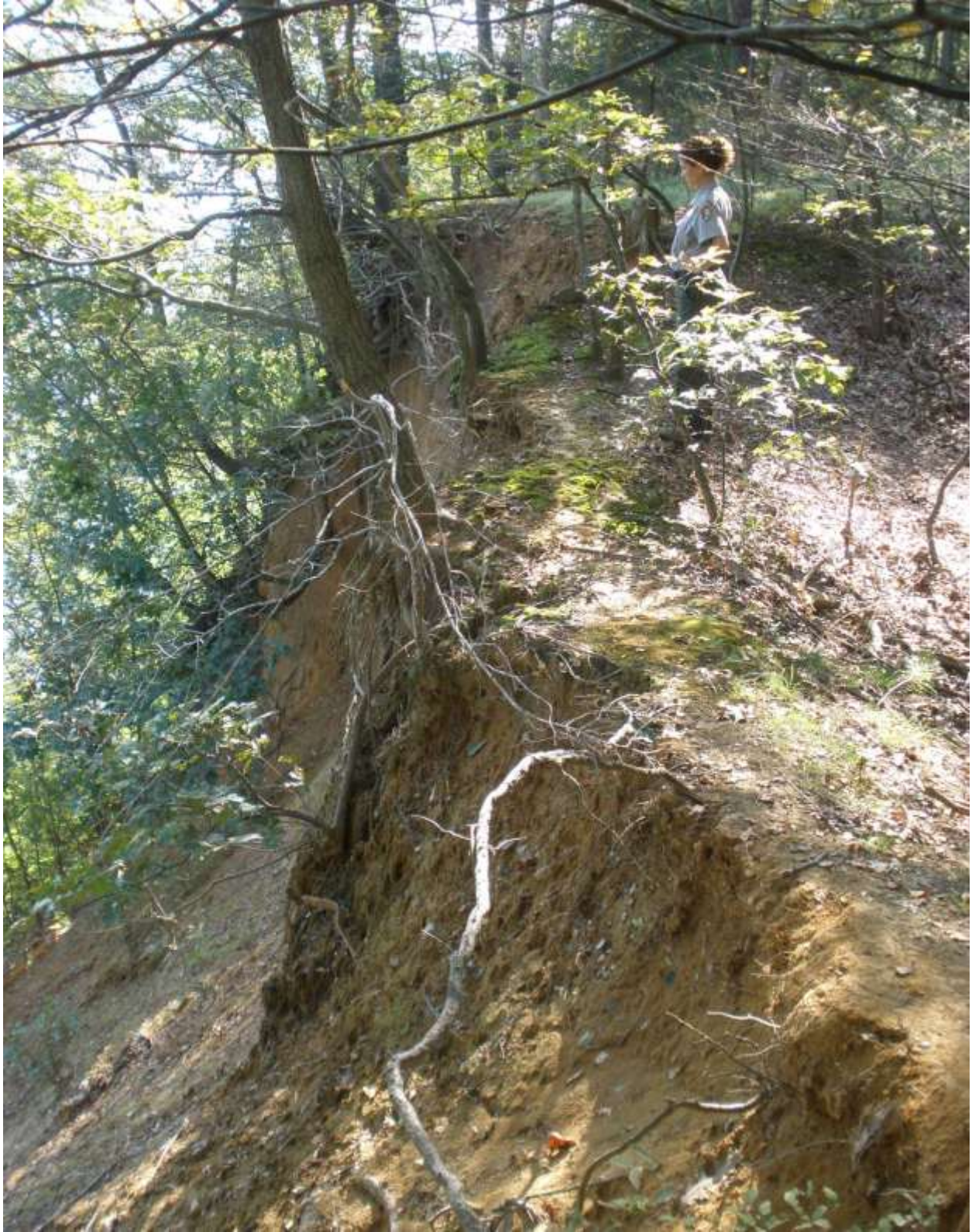
Photo of a near-vertical face at the top of the bluff. Failure and slumping of this area is inevitable. When that happens, the edge of the bluff will have migrated some distance to the right of the area shown in the photo.
