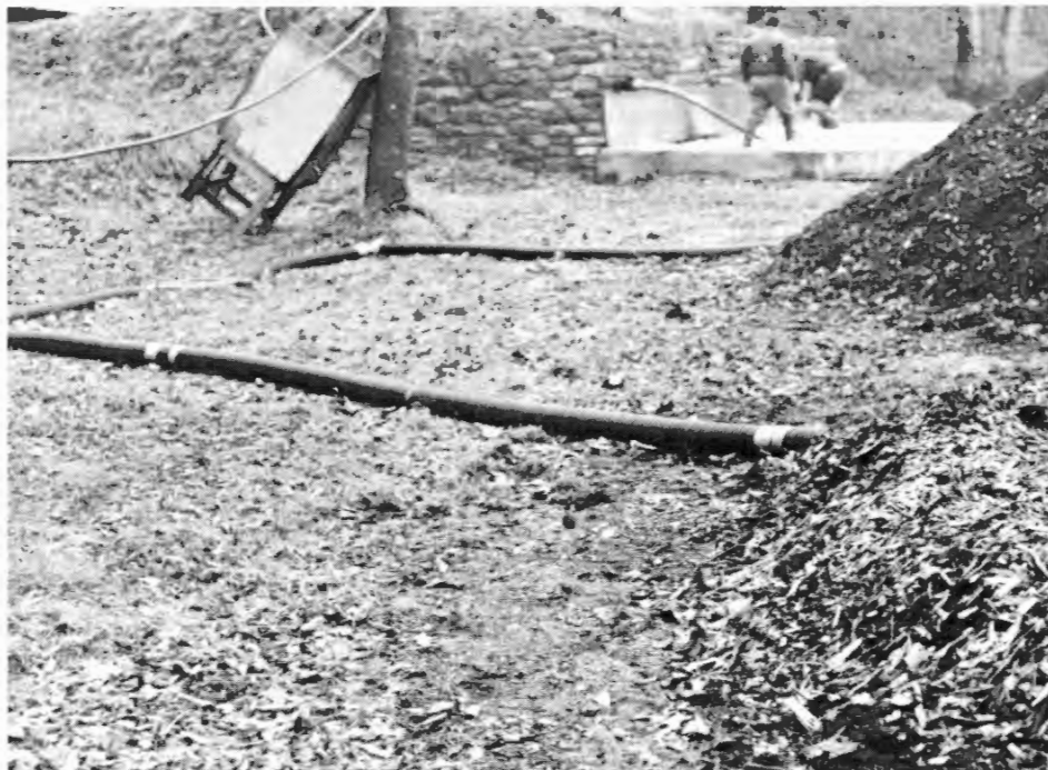
Perforated piping and the mattress are in place at the right, while the solid (non-perforated) piping connects perforated piping of the pile.
