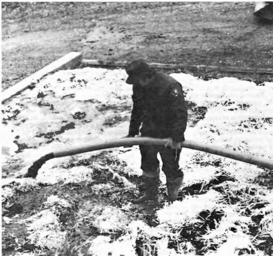
Gravity flow from an elevated storage tank allows for efficient emptying of the tank. The absorptive organic mixture of shredded waste paper, compost, wood chips, leaves and sawdust effectively absorbs the liquid waste. Absorption will proceed for about 30 minutes.
