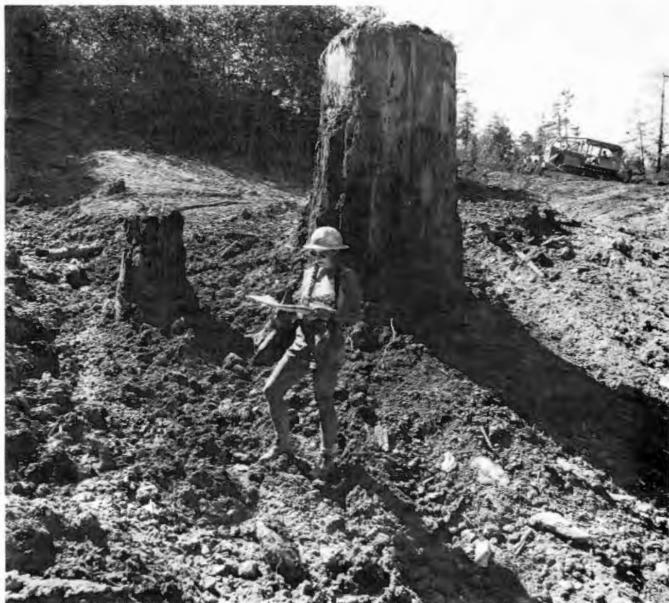
An unearthed redwood stump, its 14-foot crown marking the level of an old logging road, is a measure of the recontouring needed to control erosion and stabilize a scarred landscape in Redwood Creek watershed. Park geologist Terry Spreiter directs operations with an eye toward relocating original stream channels that may carry 20 times their normal sediment load.
