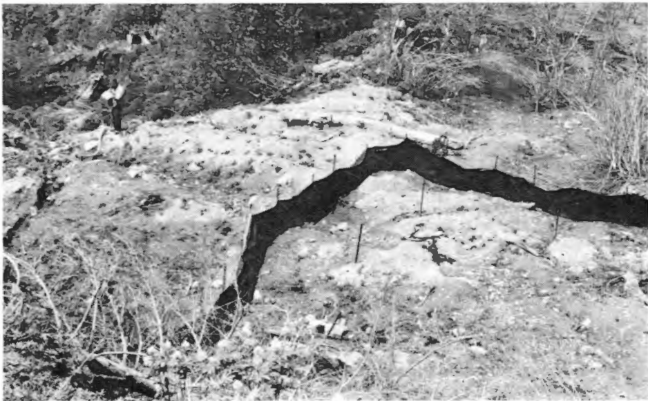
Looking downslope at Check Dam #4 on USFS 4045D road with wet slope and May 1983 slide in the distance. Dam #4 stored no sediment and basically no material was transported out of the upslope scar from the December 1981 slide. Streamflow out of the old slide scar is diverted by road to the right in the photo, only to cross the road and travel downslope, causing increased soil saturation in the vicinity of the new slide.
