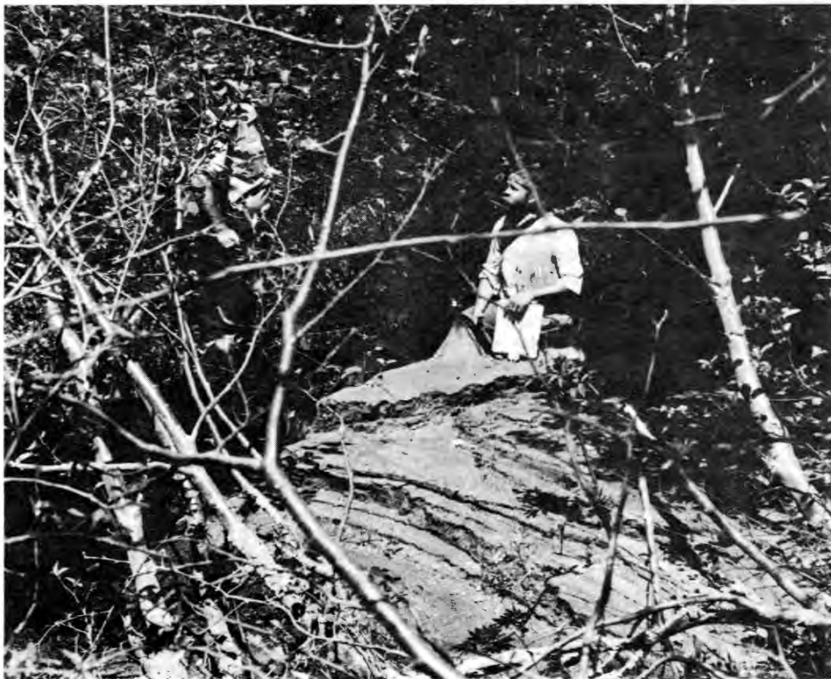
The lowest sediment storage structure installed by Forest Service personnel was this check dam made of chain-link fence and a filter fabric. The dam, (#1) built next to a large windfall log, collected and stored sediment through much of the 1982-83 winter after which the channel changed course (braided), leading to a lowering of the baseland. Approximately one half to one third of the stored sediment was eroded and transported downslope.
