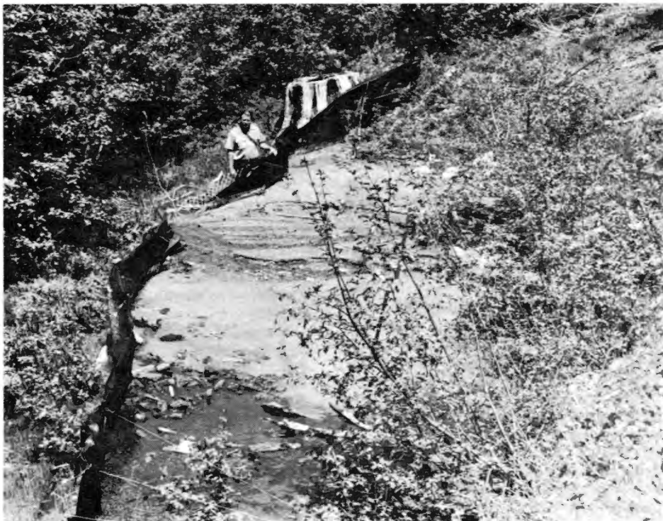
The next higher dam, (#2), built by the Forest Service, functioned well until May 1983 when a rotational slide occurred, resulting in a mudflow down the channel and causing failure of check dams Nos. 2 and 3 (see next photo). The No. 2 dam currently has no available future storage, so it will only route sediment through or over the dam. Dam No. 2 has the potential of failing in the same manner as Dam No. 1 and transporting stored sediment toward Lake Creek.
