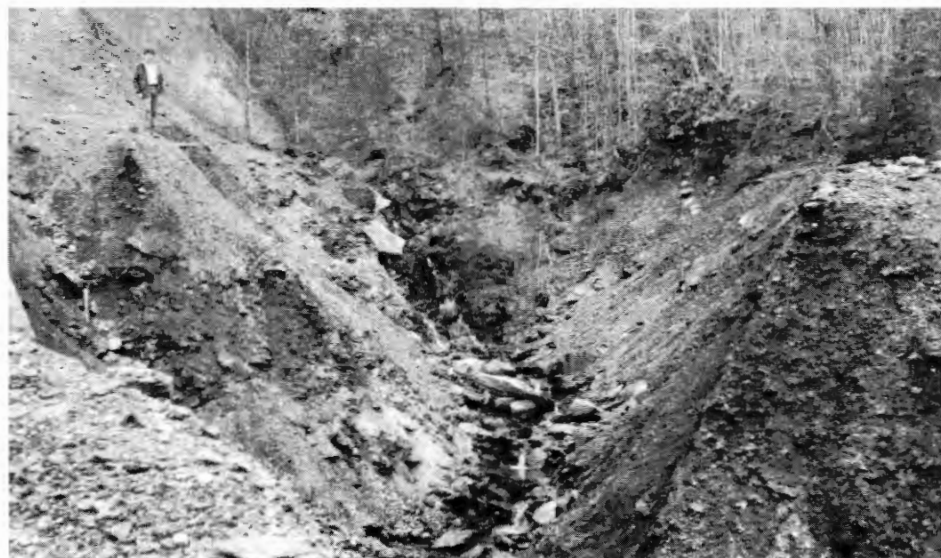
Eroding mine spoil embankment dwarfs the human figure in the gorge area of Big South Fork National River and Recreation Area.
