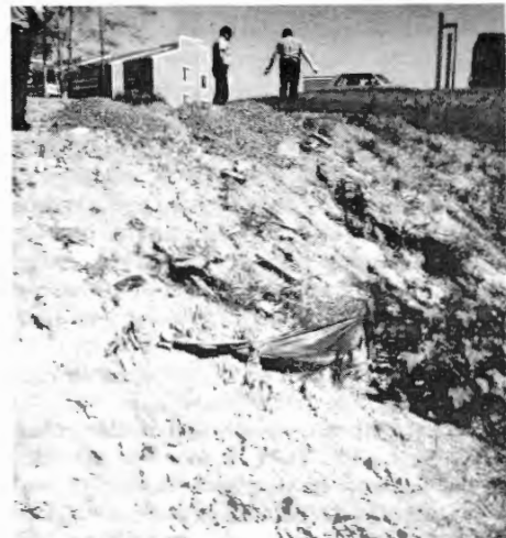
Figure 2. Housing construction can cause erosion, which flows as sediment downstream during storms. This eroded site is only about 100 meters from the park boundary at Richmond National Battlefield Park.
