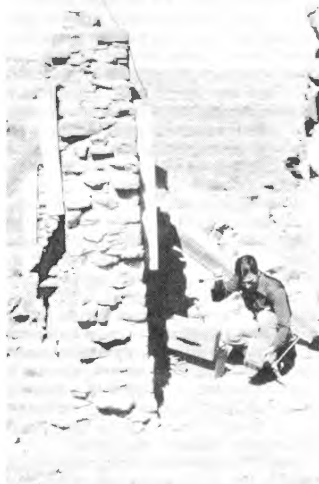
Propping and bracing of a wall at Casa Chiquita after the wall's response to energy inputs. Ken King checks the new readings.
