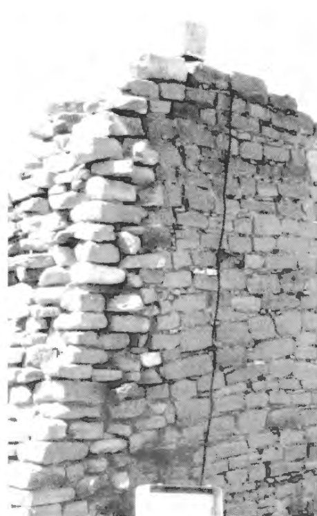
Seismometer mounted on a typical Chaco wall is employed to determine the wall's vibrational response to energy inputs.
