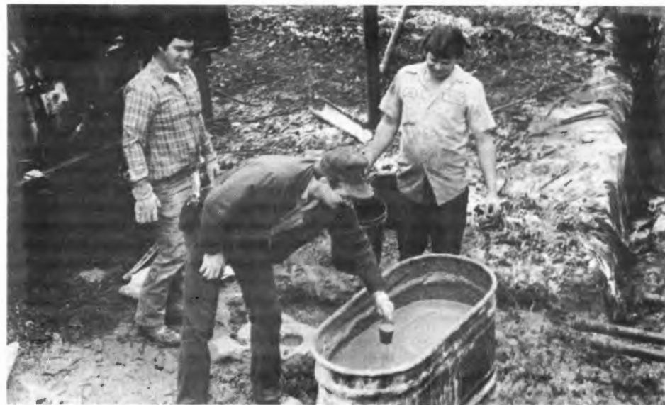
Mammoth Cave Ranger Henry Holman pulls sample of cement used to set surface marker.
