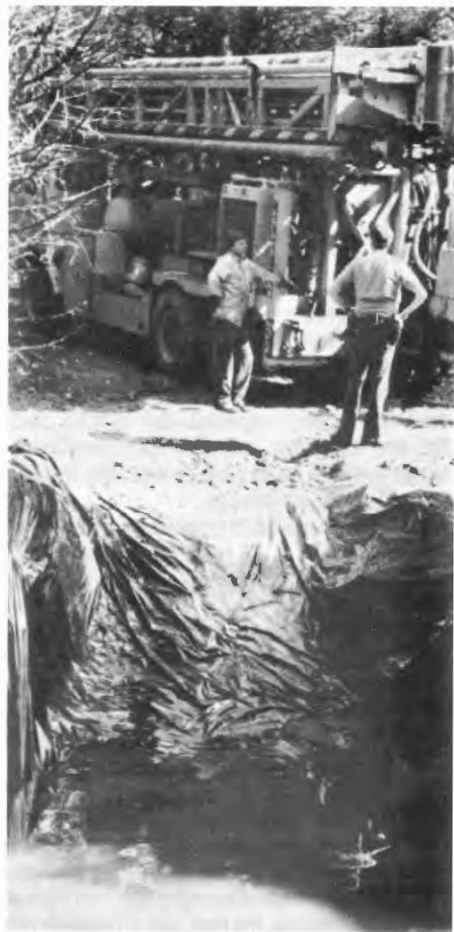
Plastic lined pit in foreground catches excess cement or groundwater.
