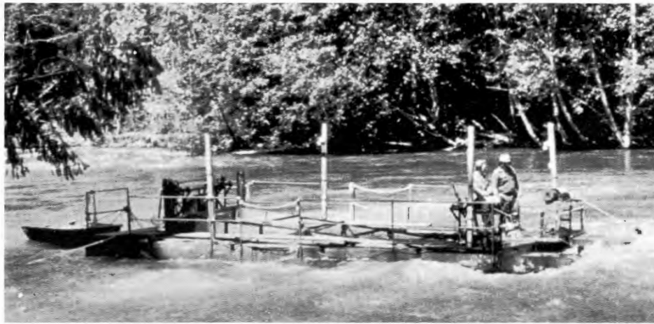
Inclined plane smolt trap operates below the Elwha dam to sample smolt survival.
