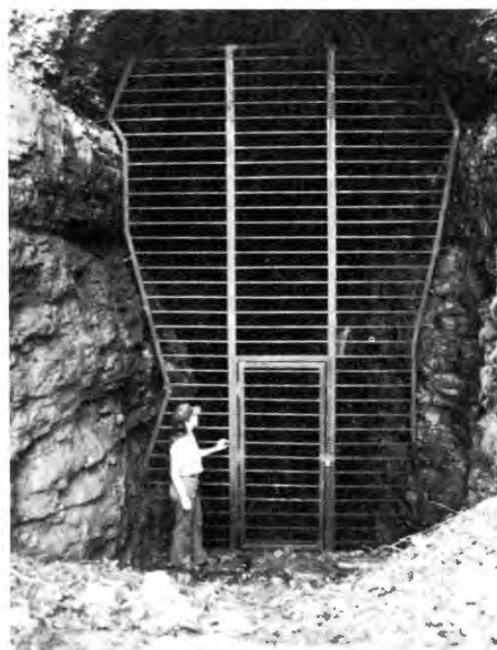
Natural Resource Specialist Margaret Weesner looks at a "bat gate" installed at the now reclaimed Kaymoor Mine. Photo by Margaret Weesner.
